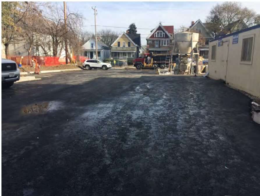
Photo 10: Asphalt binder course installed in north and northeast portion of Site on November 13, 2017. View looking to east.
