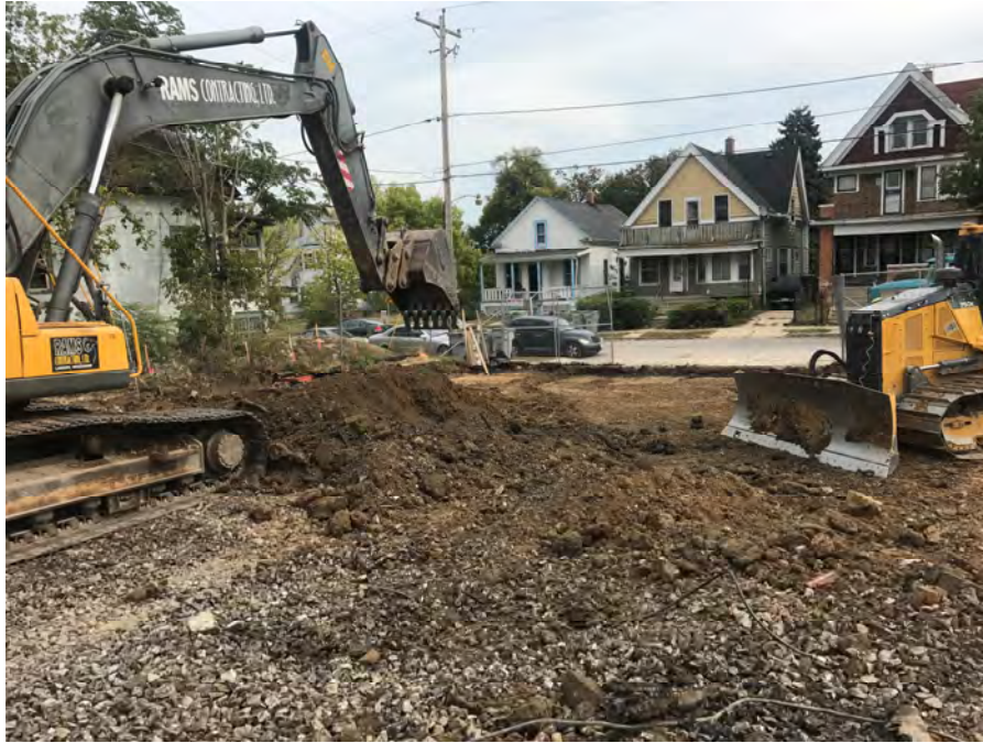
Photo 1: Parking lot subgrade removal in progress in northeast portion of Site on October 2, 2017. View looking to northeast.
