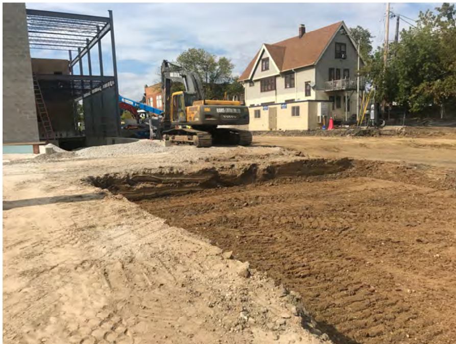
Photo 4: Parking lot subgrade removal (including area for pervious pavers and underlying storm water retention) in north-northeast portion of Site on October 3, 2017. View looking to northwest.
