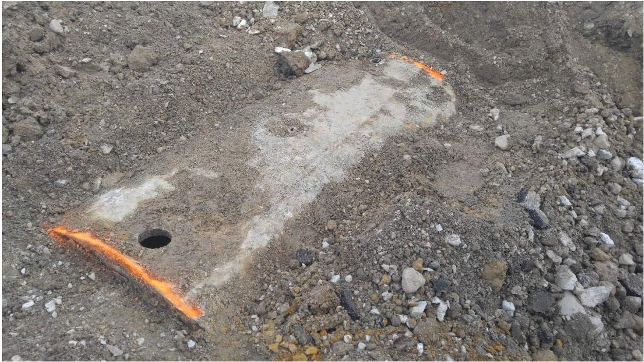
ONE THOUSAND (1,000) GALLON WASTE OIL UNDERGROUND STORAGE TANK (UST) DURING EXCAVATION
