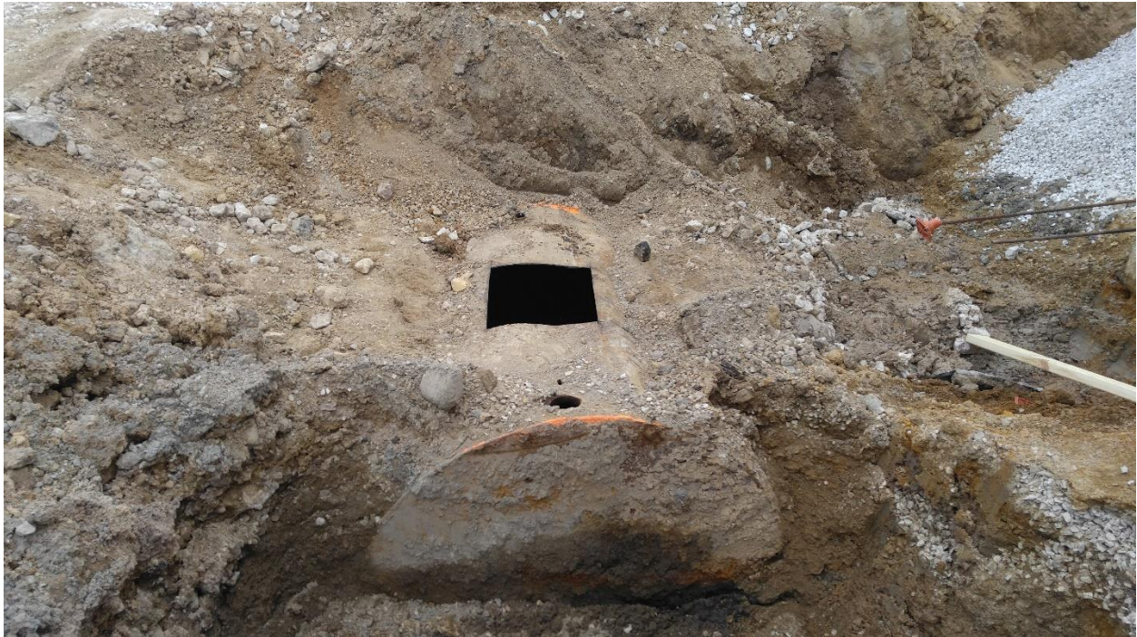
ONE THOUSAND (1,000) GALLON WASTE OIL UST PRIOR TO REMOVAL
