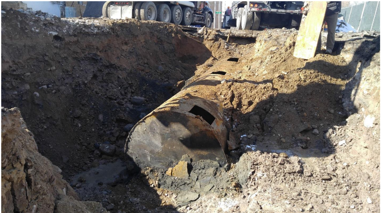
FOUR THOUSAND (4,000) GALLON UST PRIOR TO REMOVAL LOOKING WEST-SOUTHWEST
