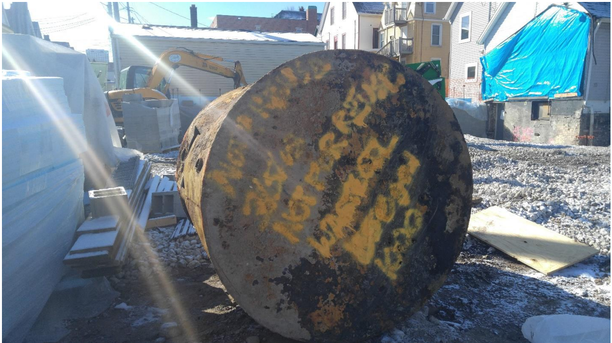
ONE THOUSAND (1,000) GALLON WASTE OIL UST SUBSEQUENT TO REMOVAL AND LABELING
