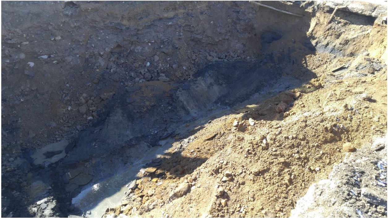
EXCAVATION LIMITS LOOKING SOUTHWEST SUBSEQUENT TO THE REMOVAL OF THE FOUR THOUSAND (4,000) GALLON UST
