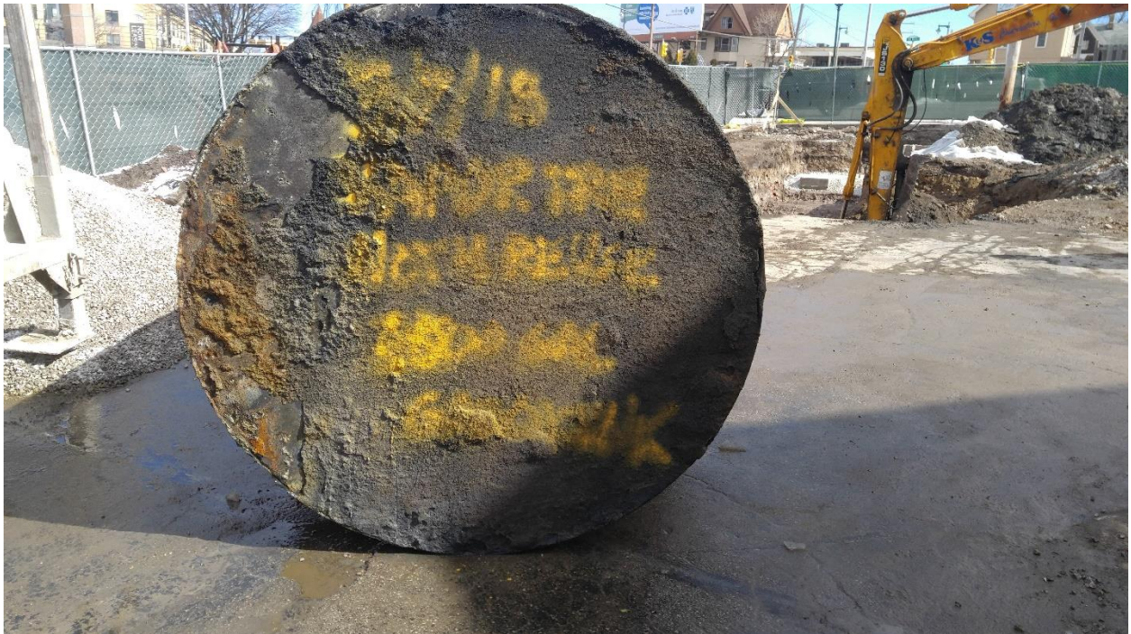
FOUR THOUSAND (4,000) GALLON UST SUBSEQUENT TO REMOVAL AND LABELING
