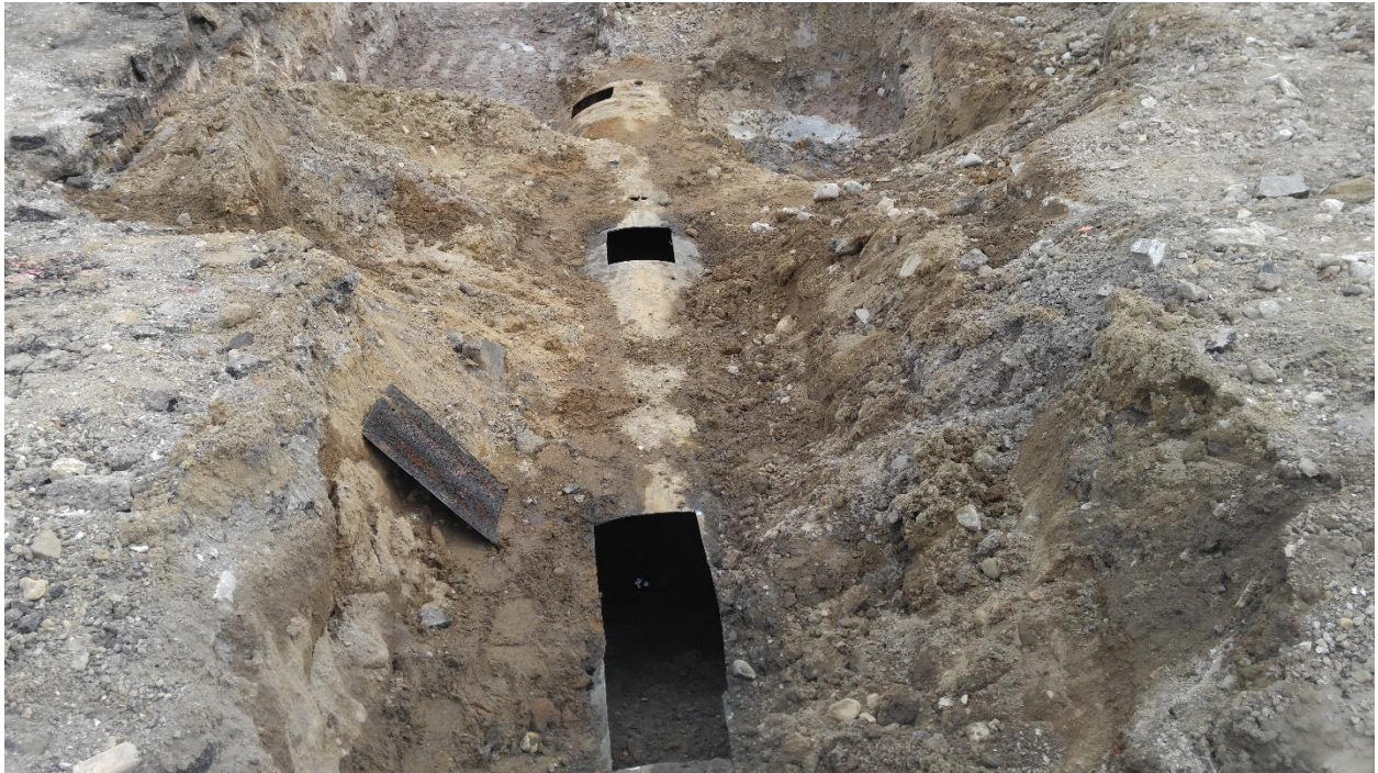
FOUR THOUSAND (4,000) GALLON UST DURING EXCAVATION LOOKING EAST
