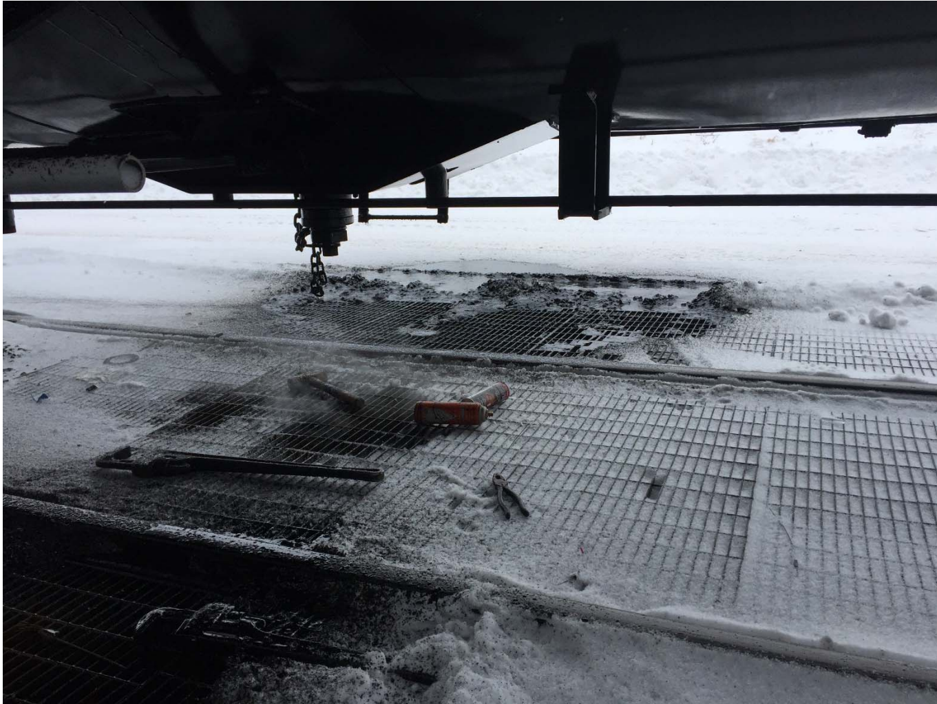
Photo 5: Looking west at the three “track pan” containments underneath the railcar on Track 3.
