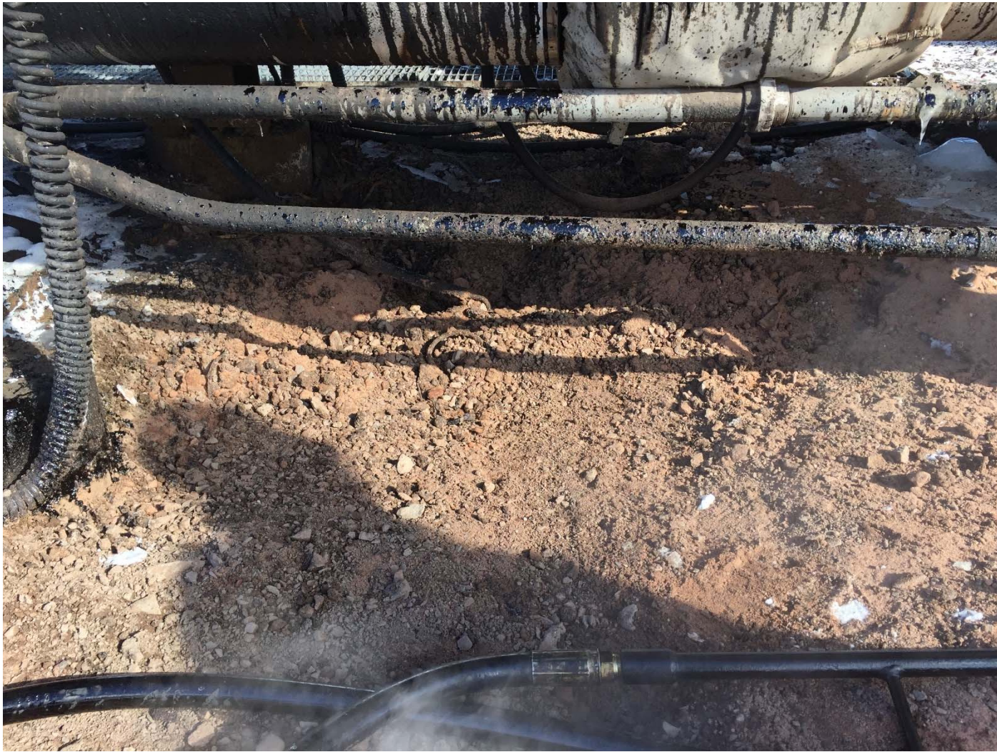
Photo 10: Looking east at the excavated affected area.
