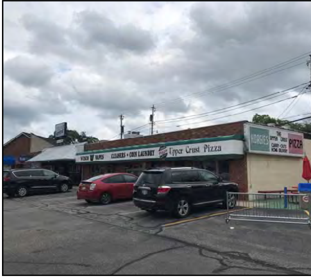
Photograph 1 - The subject property is located at 249-261 East Hampton Avenue in Milwaukee, Wisconsin. The subject property currently contains a commercial shopping center and associated parking lot.
