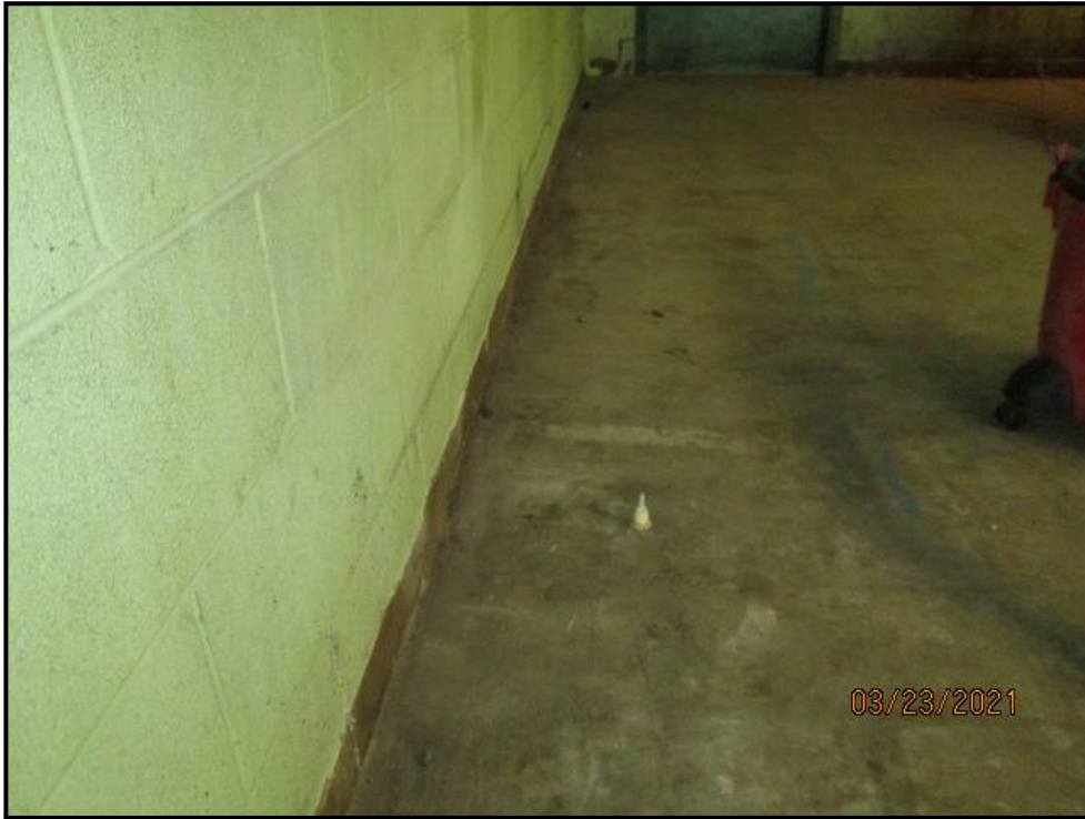
View of PFE- 1(FLC), viewing West.
