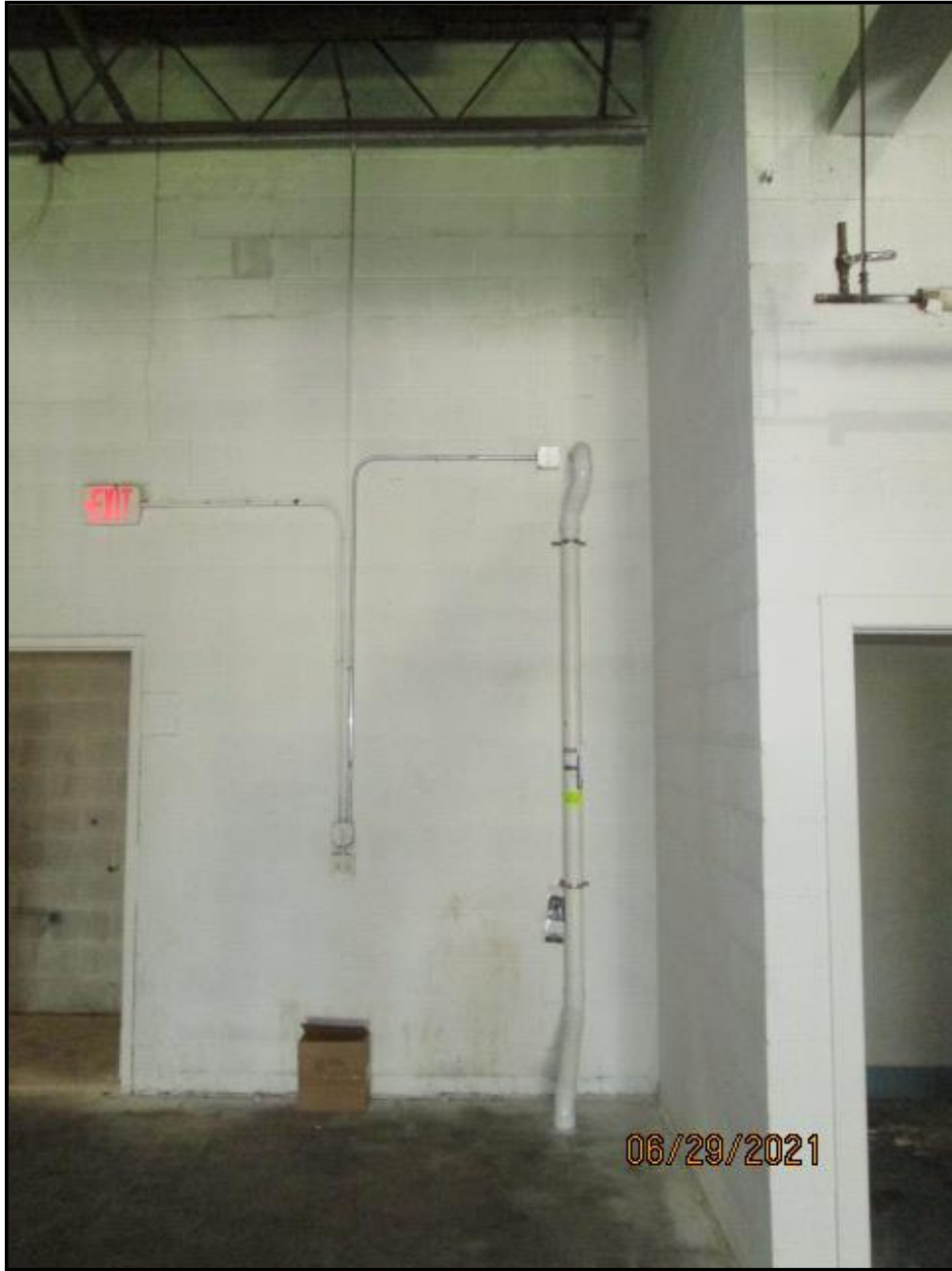
Interior completed VMS (FLC), viewing North.
