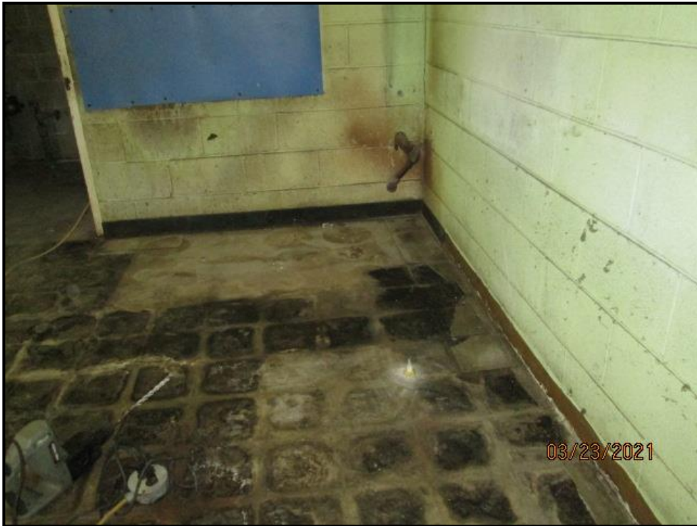
View of PFE-2 (FLC), viewing West.
