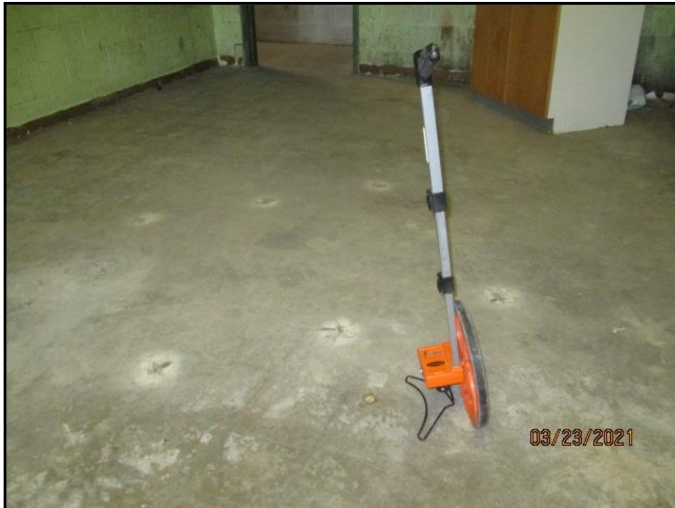
Former location of Dry Cleaner Machine (Former Lakeside Cleaners) and PFE-6, viewing North
