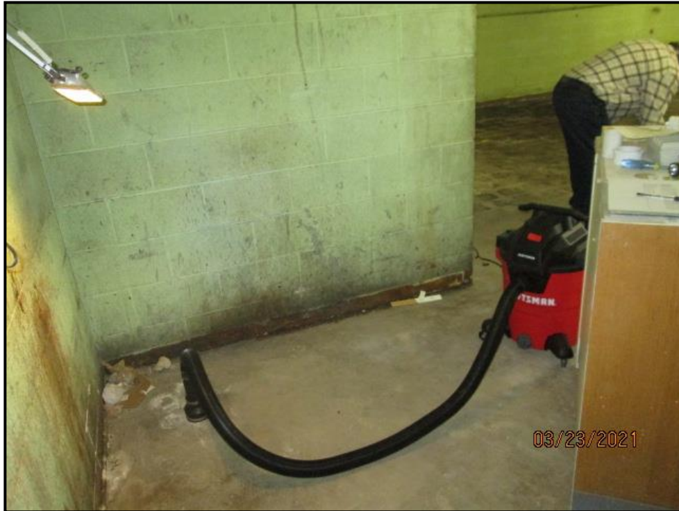
3.5" Extraction Hole with shop vac (same hole for VMS), viewing North.
