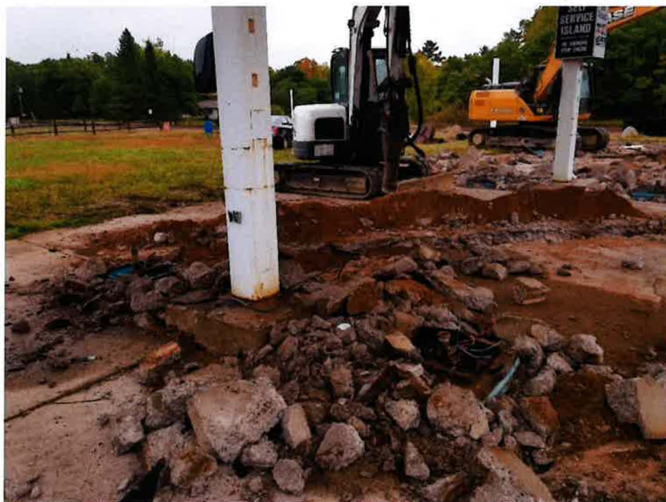
PHOTOGRAPH OF DISPENSER AREA
