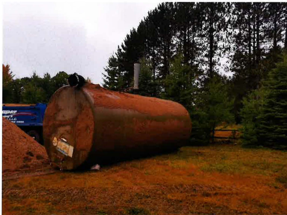
PHOTOGRAPH OF WESTERN 10,000-GALLON GASOLINE UST
