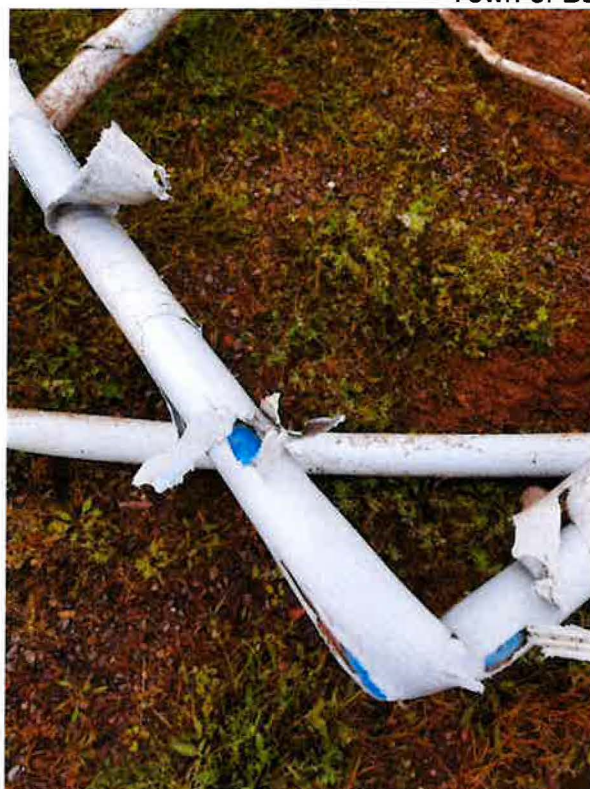
PHOTOGRAPH OF THE REMOVED DOUBLE WALL PIPING
