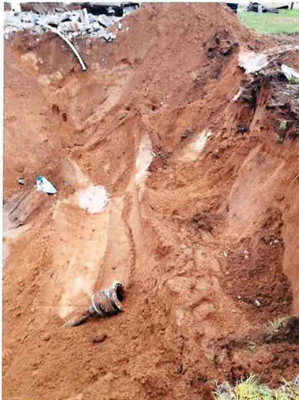
PHOTOGRAPH OF EXCAVATION VIEWING SOUTH TO NORTH
