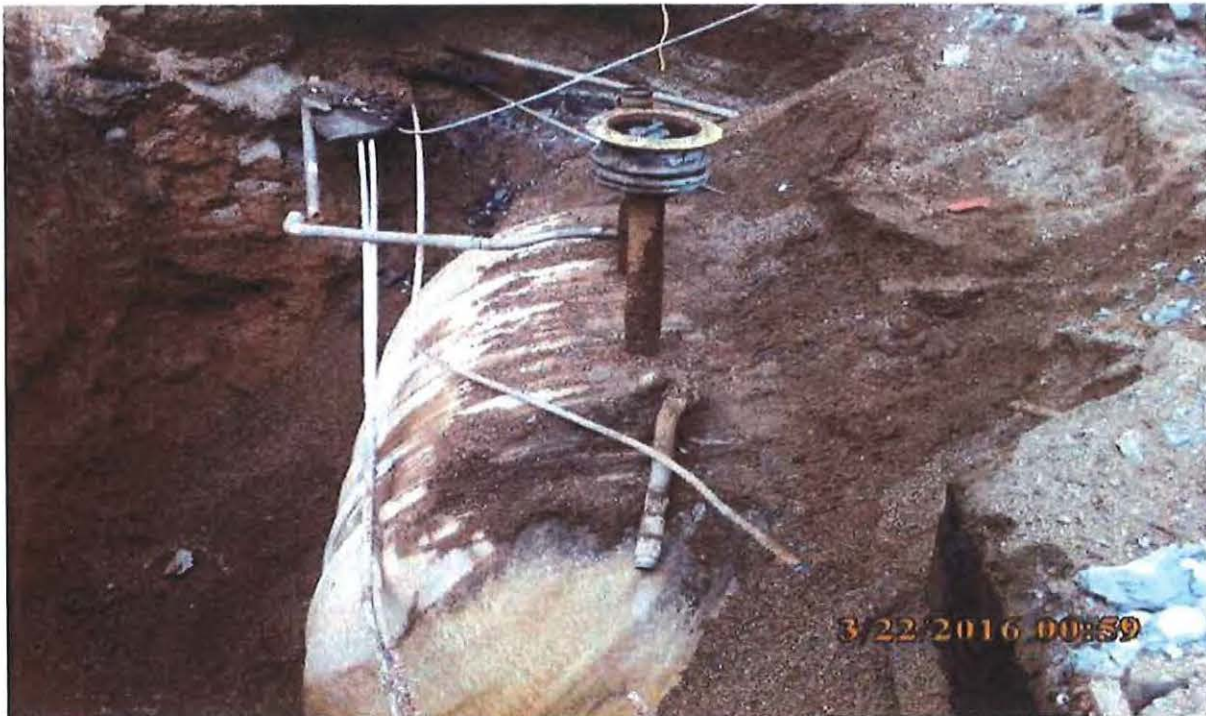
PHOTO 1 - PHOTOGRAPH OF THE 4,000-GALLON GASOLINE UST
