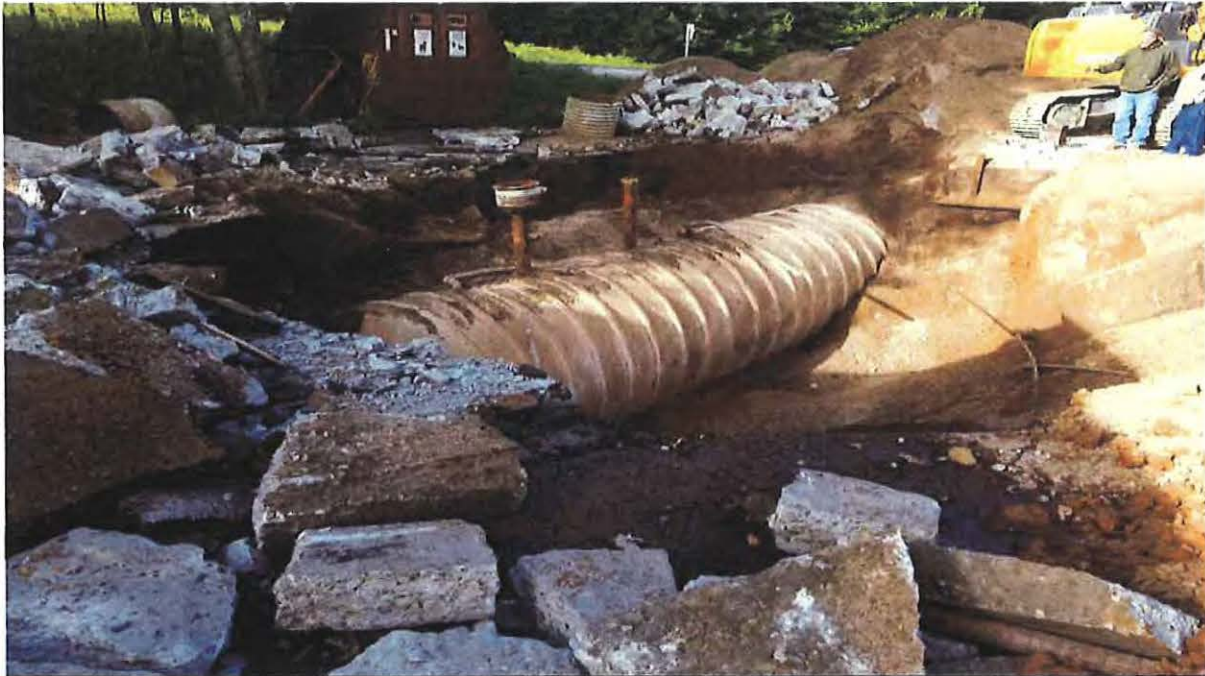
PHOTO 3 – PHOTOGRAPH OF THE 10,000-GALLON UNLEADED GASOLINE UST
