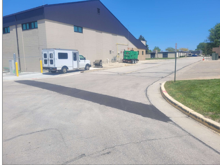
Title: Southwest Corner Building 522
