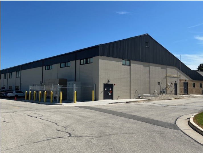
Title: Building 522 Southwest Corner
