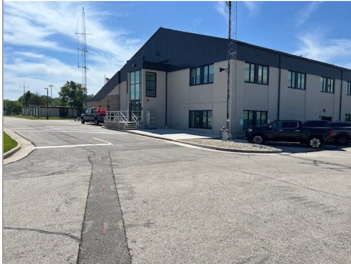
Title: Building 522 Northwest Corner
