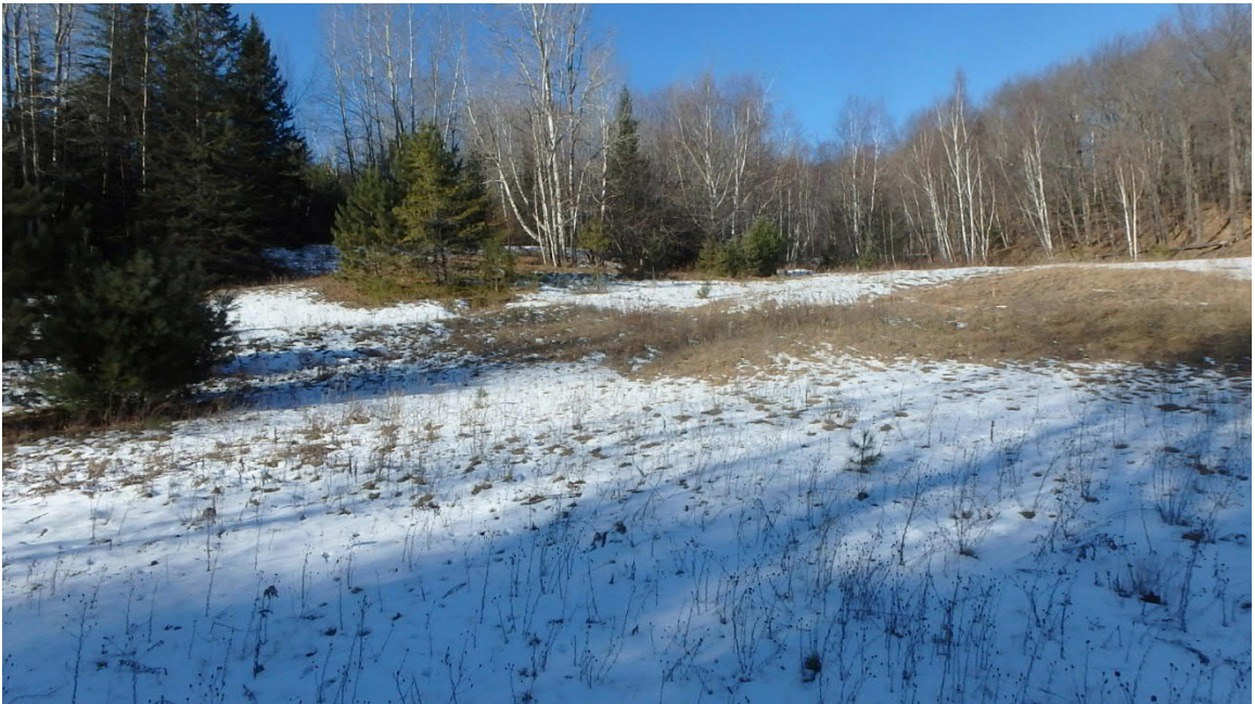
Photo PC030053- Looking west at the area of the proposed parking lot and pit toilet of the trailhead project.
