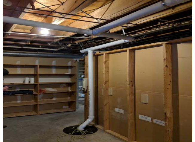
#8: View of completed pick-up point in northeast corner of basement.
