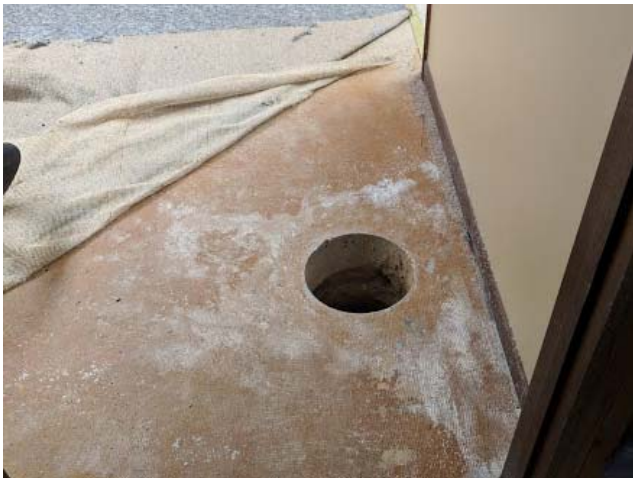
#3: Pick-up point installation through the slab exposing sub-slab materials.
