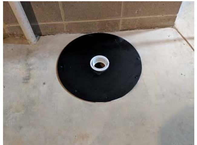
#4: Pick-up point installation sealed to concrete slab.
