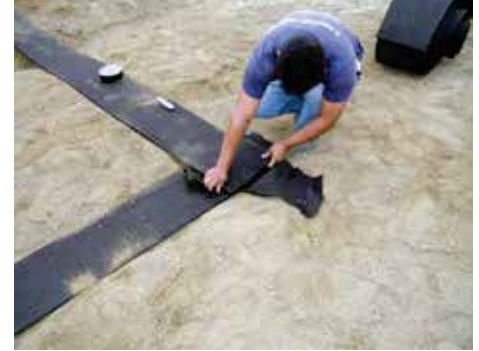
GEOVENT™ allows for ease of installation directly on the subgrade, eliminating the need for costly and labor-intensive trenching.
