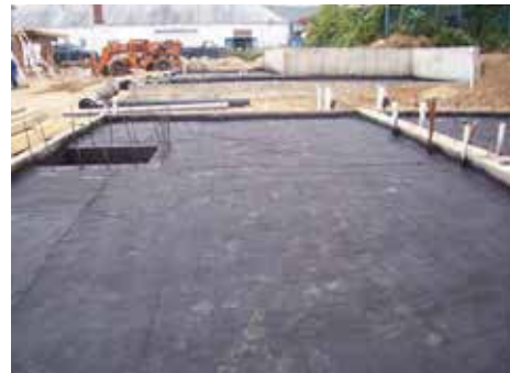
ULTRASHIELD™ G-1000 is a needle-punched, non-woven geotextile with superior tensile strength and puncture resistance.
