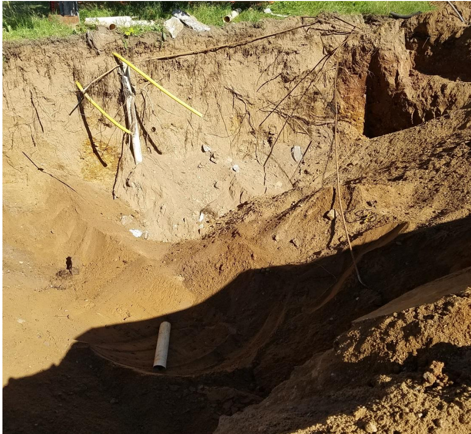
PHOTOGRAPH OF THE UST EXCAVATION
