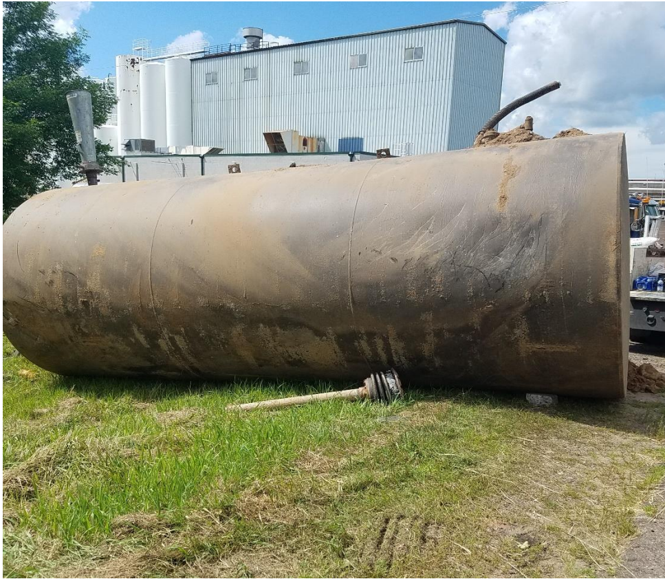
PHOTOGRAPH OF 10,000-GALLON DIESEL TANK
