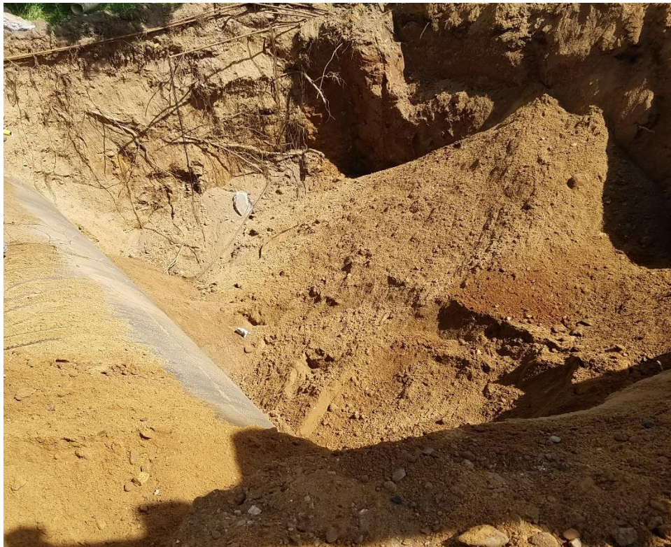
PHOTOGRAPH OF EXCAVATION BENEATH THE 10,000-GALLON DIESEL TANK
