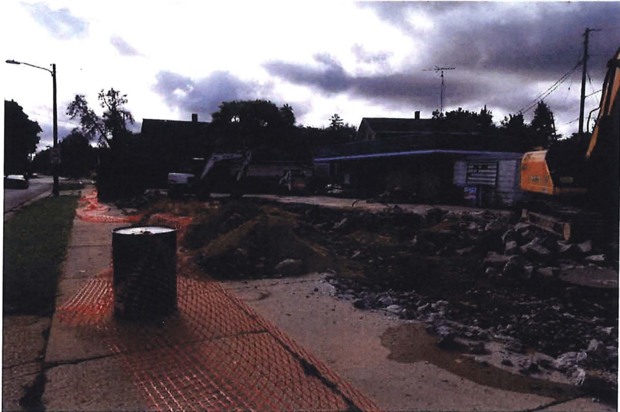
PHOTOGRAPH OF THE ARE OF THE FORMER DISPENSERS AND CANOPY
