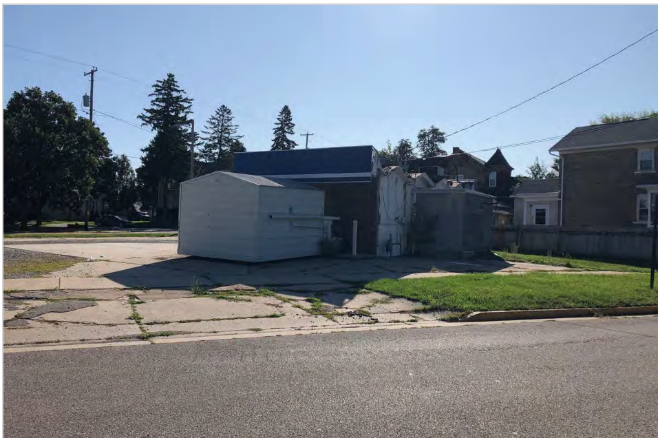
3) View of the subject property from the south
