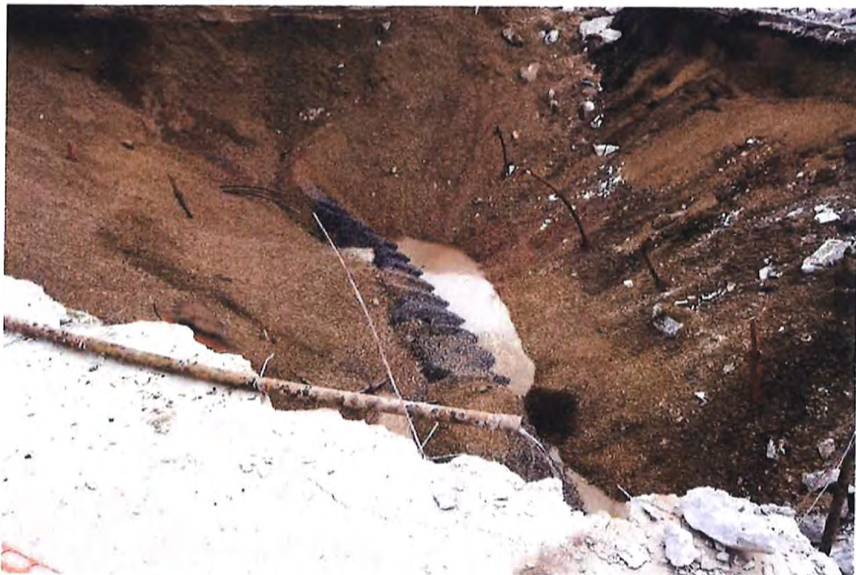
PHOTOGRAPH OF EXCAVATION AFTER THE 10,000-GALLON TANK REMOVAL
