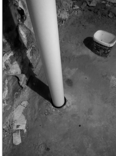
Title: Vapor Pickup Point showing Floor Seal
