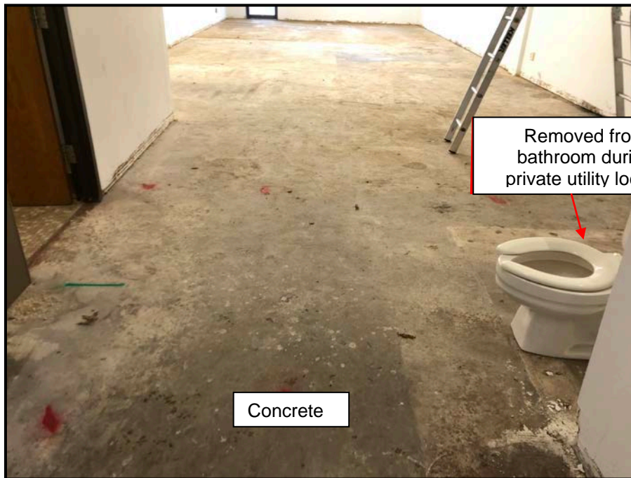
View of the interior of source unit and typical concrete floor to be maintained, facing east.
