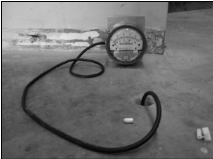
View of a manometer reading at SS-1 showing negative pressure of 0.2 inches of water.
