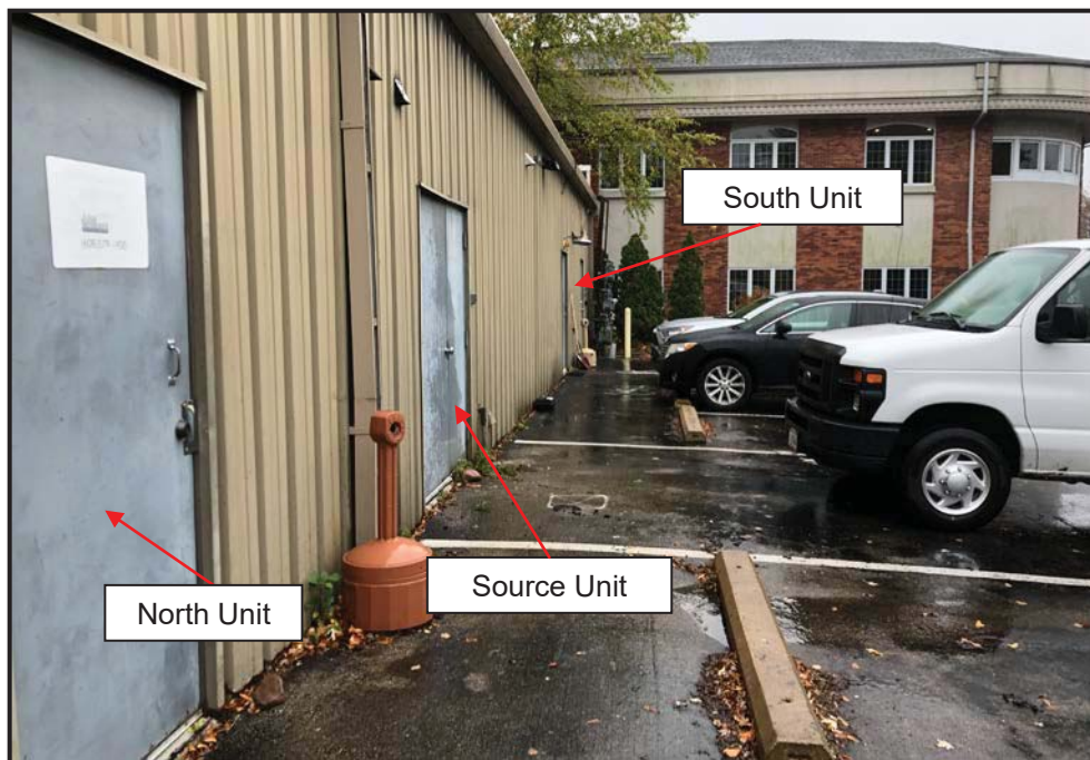
View of the back of the shopping center building, facing southwest.
