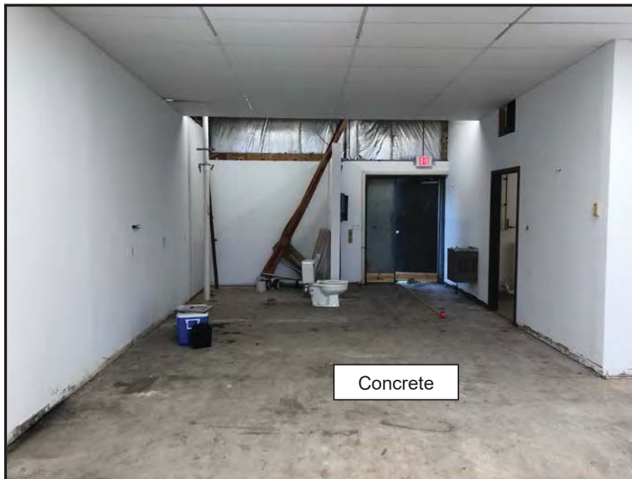
View of the interior of source unit and typical concrete floor to be maintained, facing west.
