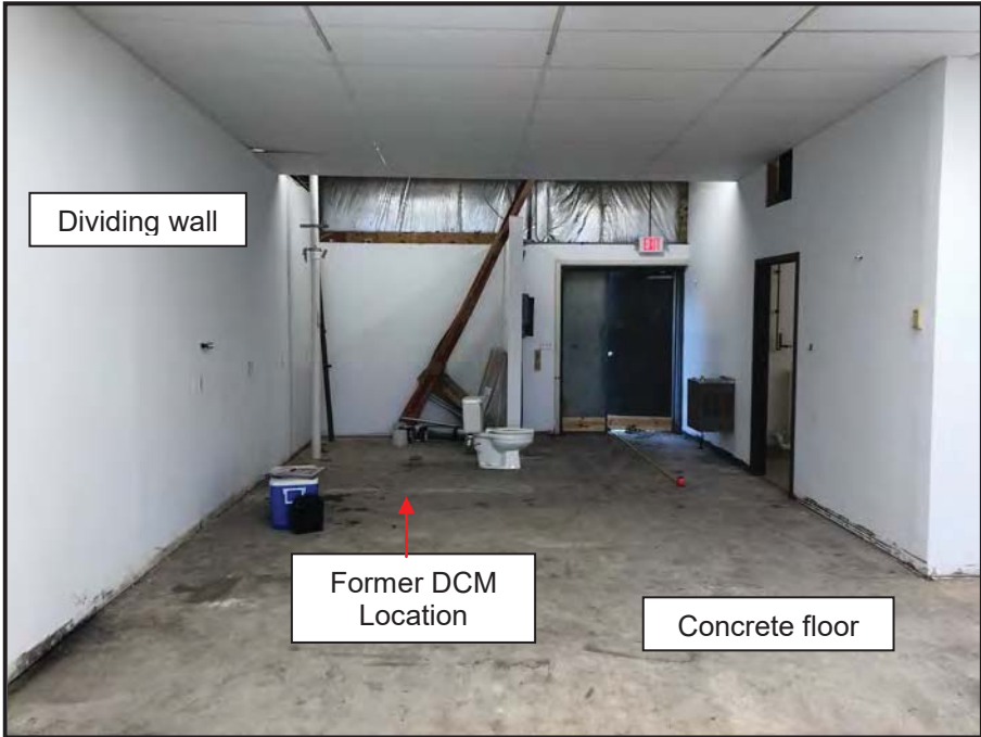
View of the interior of source unit and concrete floor that will act as a performance cap, facing west.
