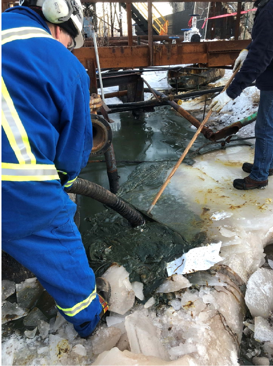
Photo 3: Looking south at the recovery efforts. Note the thick layer of ice present underneath the released #6 fuel oil.
