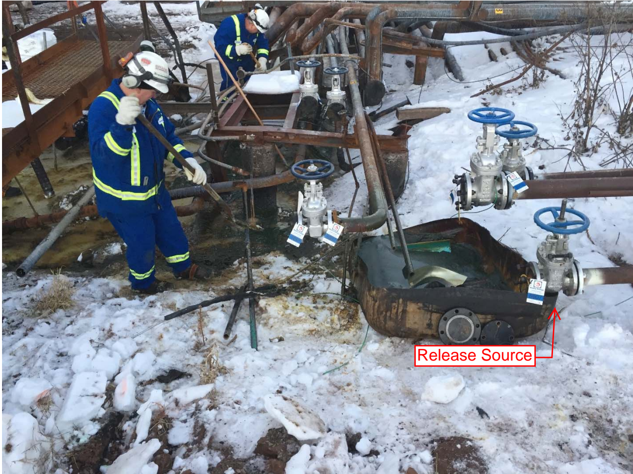
Photo 2: Looking east at the release site while cleanup efforts are ongoing. Operators used shovels and squeegees to move the product to a vacuum truck hose so it could be recovered. The cold air temperatures thickened the product to a pudding-like consistency.
