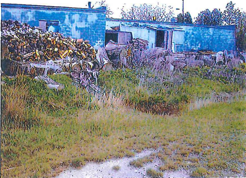
View to the southeast, west side of 8655 N. 43 rd Street. Discharge area visible in the center of the photo.
