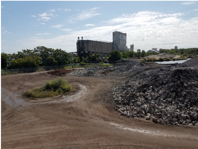
3. view of some vegetation and process demolition debris, looking east/southeast
