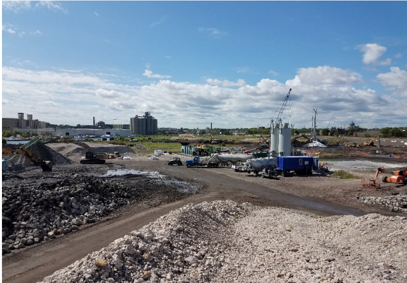
1. View of demolition debris processing and active remediation, looking south
