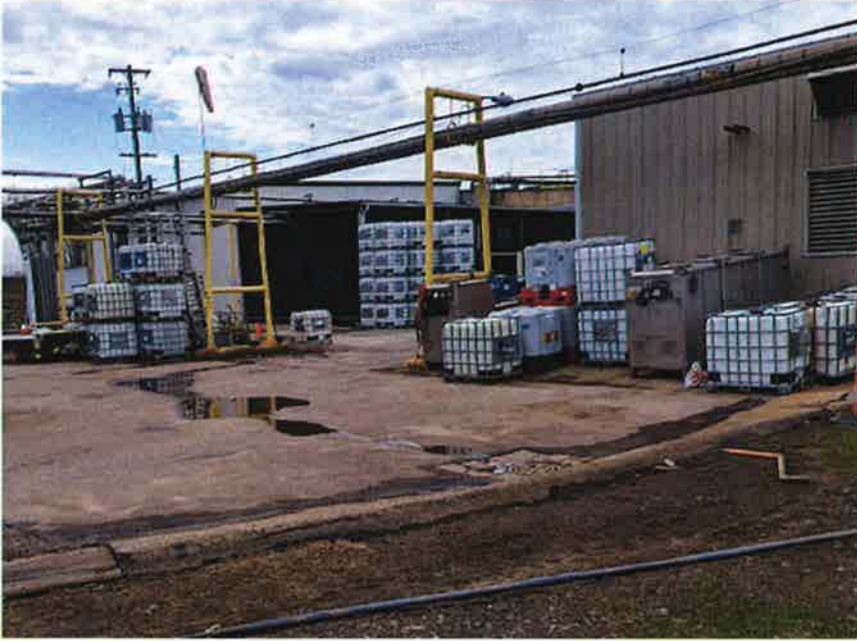
Pic 5 – Spill containment area\Hold and Test containment area
