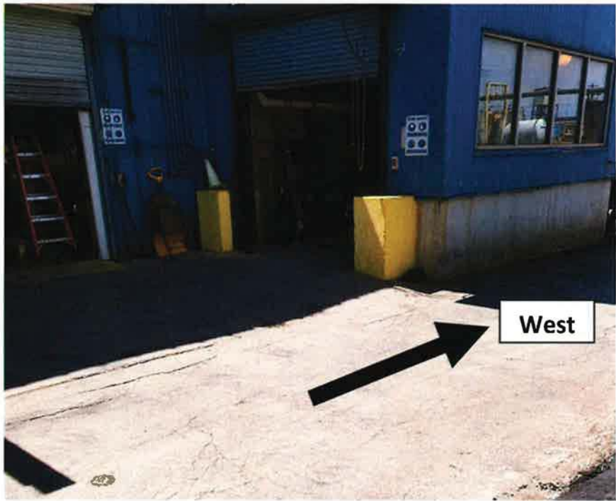
Pic 2 - Bldg 52, 5228's room to the North of the building. The spill drained to the West into our Hold and Test containment area
