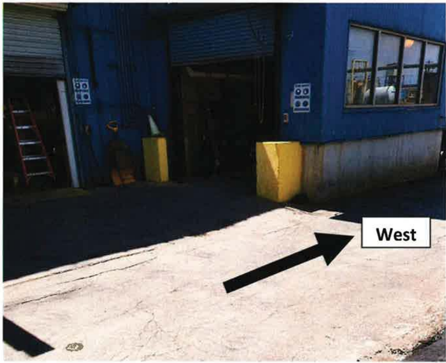
Pic 2 - Bldg 52, 5228's room to the North of the building. The spill drained to the West into our Hold and Test containment area
