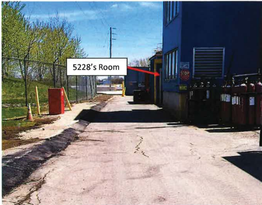
Pic 3 - View to the East after clean-up and gravel fill
