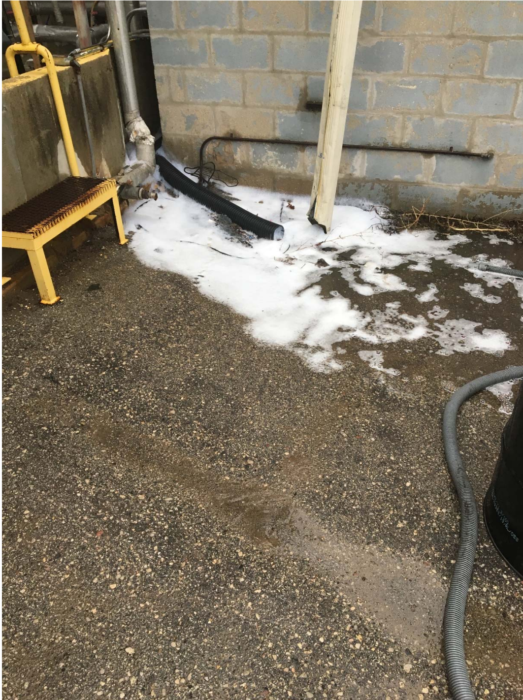
Photo showing roof drain from B18 into industrial sewer.
