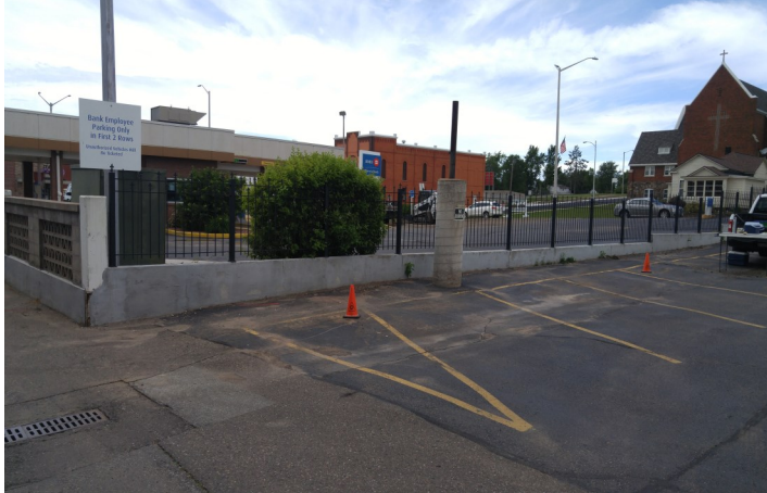
1. Photograph shows highway cones placed at the locations of SP-1 (left) and SP-2 (right) and the surrounding asphalt pavement and small retaining walls associated with the Subject Property. The photograph is taken facing to the west from the alleyway.
