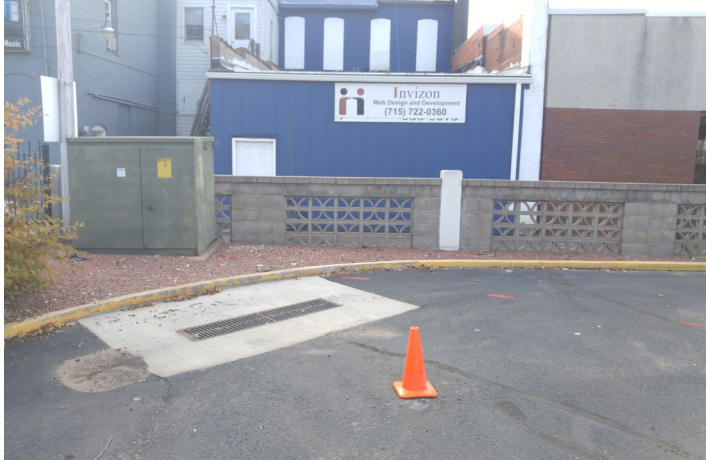
10. Photograph shows a highway cone over SP-14 and a stormwater drain.
