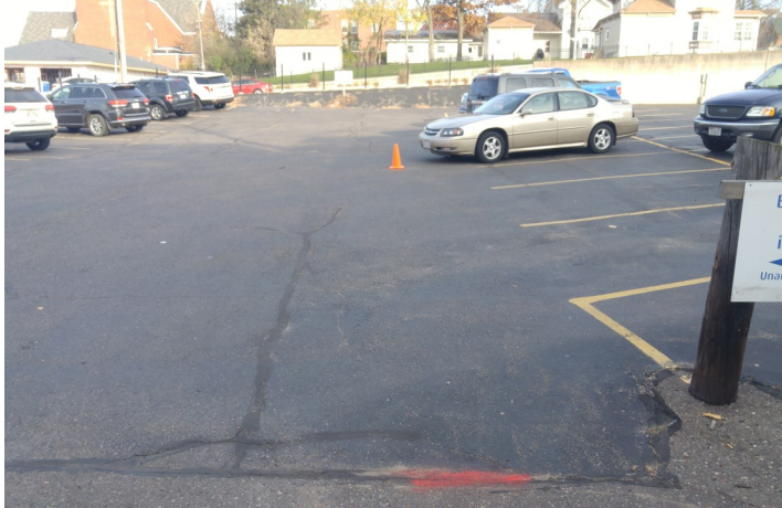
7. Photograph taken from the alleyway and facing to the north and shows the northeastern portion of the asphalt parking lot area. The highway cone is over SP-17 and SP-7 would be to the northwest of SP-17.
