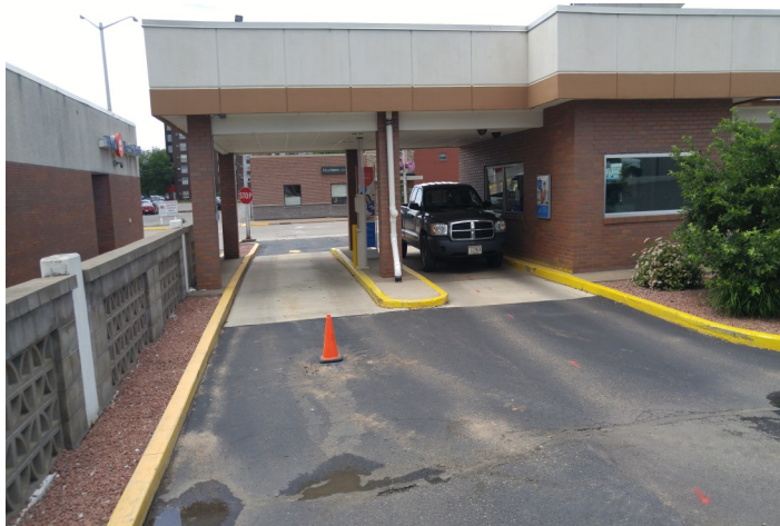
3. Photograph shows the southern drive-thru lines of the service window building and the highway cone is placed over SP-3. The photograph also shows the retaining wall along the alleyway and the asphalt and concrete pavement associated with the bank parcel.
