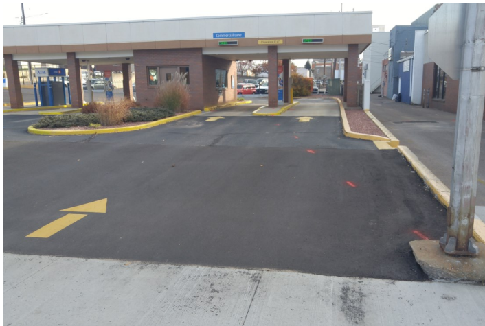
12. Photograph shows the western side of the drive-thru window building and the alleyway (right side of photo). Photograph also shows asphalt and concrete pavement associated with the bank parcel.
