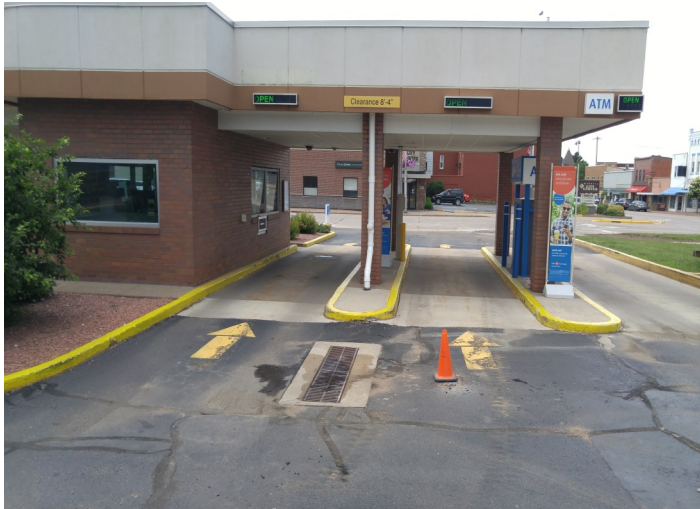
2. Photograph shows the northern drive-thru lines of the service window building associated with the BMO Harris Bank parcel. The highway cone shows the location of SP-4. A stormwater drain is located south of SP-4. SP-11 was placed in the grass area shown on the right side of the photograph. Photograph taken facing to the west.
