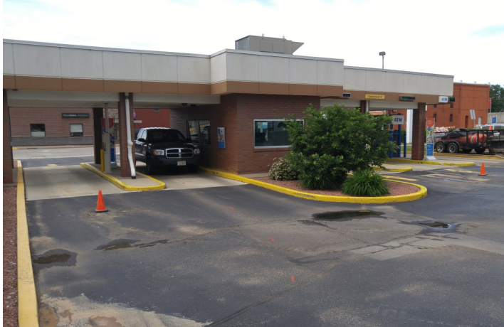
4. Photograph shows the drive-thru window building and SP-3 (left) and SP-4 (right).
