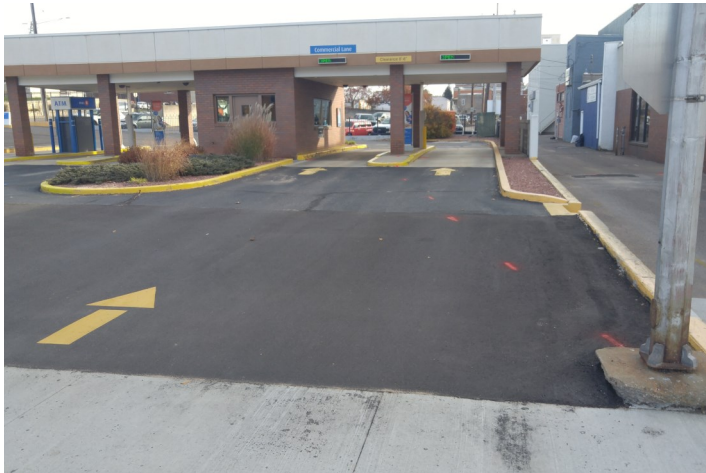
12. Photograph shows the western side of the drive-thru window building and the alleyway (right side of photo). Photograph also shows asphalt and concrete pavement associated with the bank parcel.
