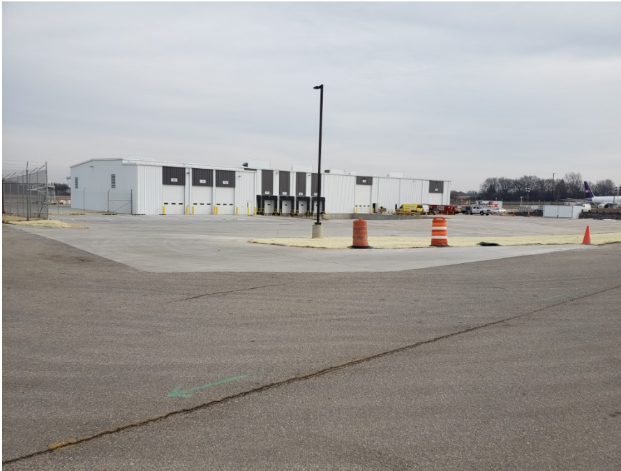
Photo 9: View of the completed building looking southeast from Bowman Street (12/15/21; 10:42)
