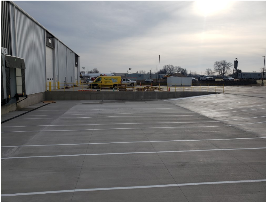
Photo 11: Loading dock area looking south (12/15/21; 10:44)
