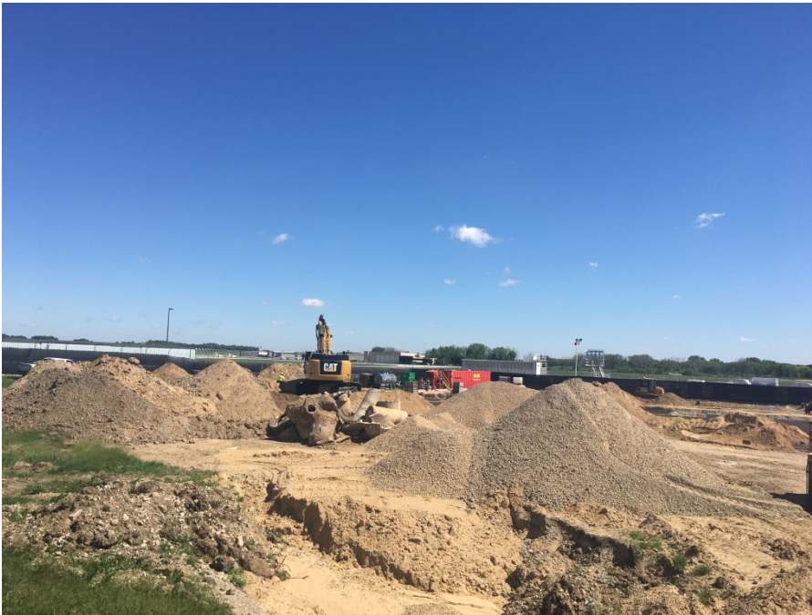
Photo 8: General site conditions, looking northeast (5/26/21; 10:26)
