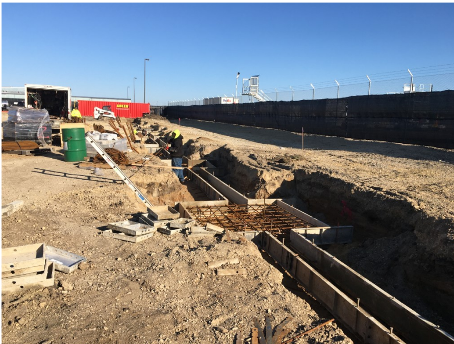
Photo 4: Building footing trench looking north (4/1/21; 08:44)
