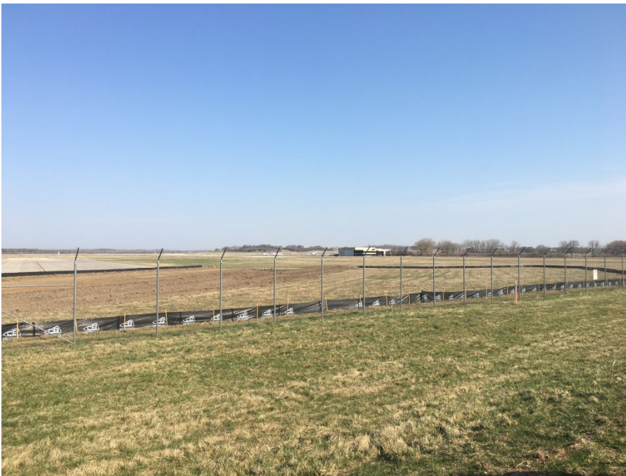
Photo 6: Soil replacement area looking north (4/7/21; 09:18)
