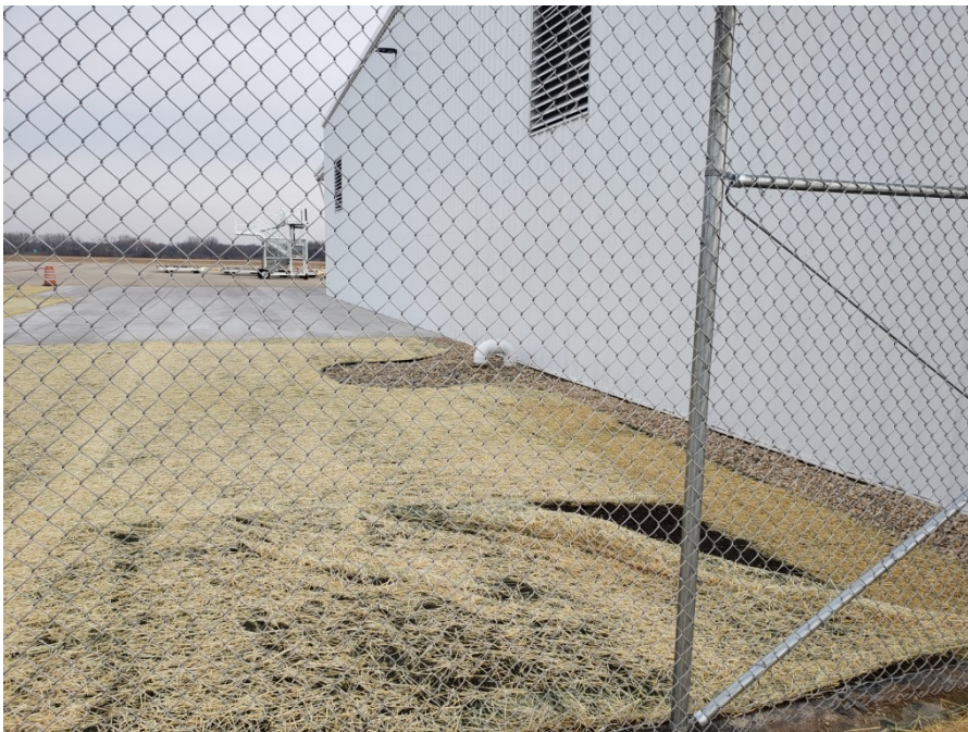
Photo 10: Landscaped area on the north side of the building looking east (12/15/21; 10.43)
