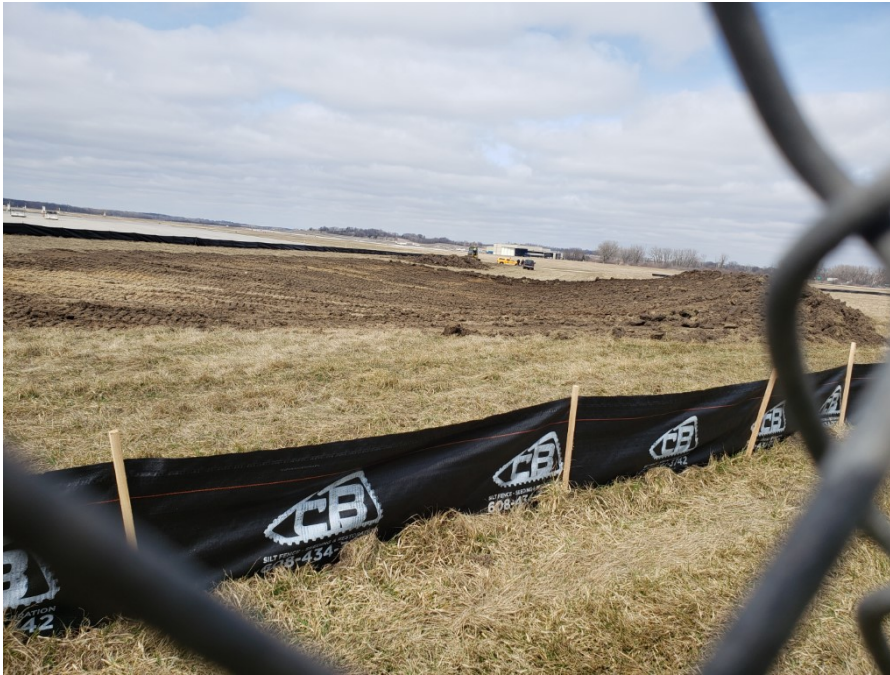
Photo 3: Soil replacement area with partially stripped topsoil, looking northwest (3/26/21; 13:39)
