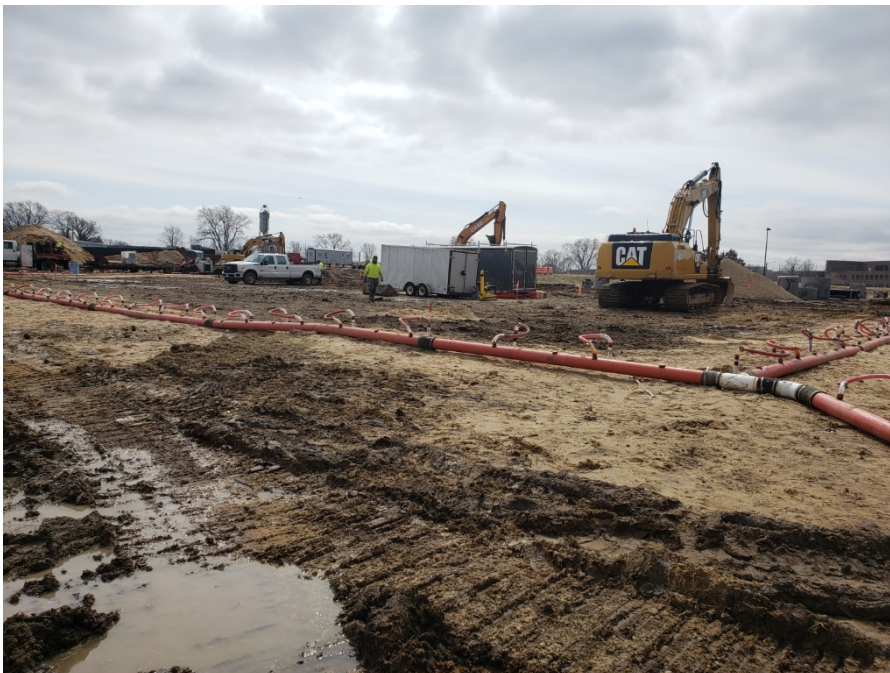
Photo 2: Dewatering system header pipes around dock excavation area, looking southwest (3/26/21; 13:27)
