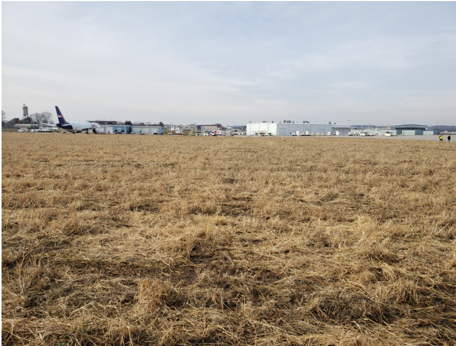
Photo 15: Soil replacement area looking west at new building (12/15/21; 11:19)
