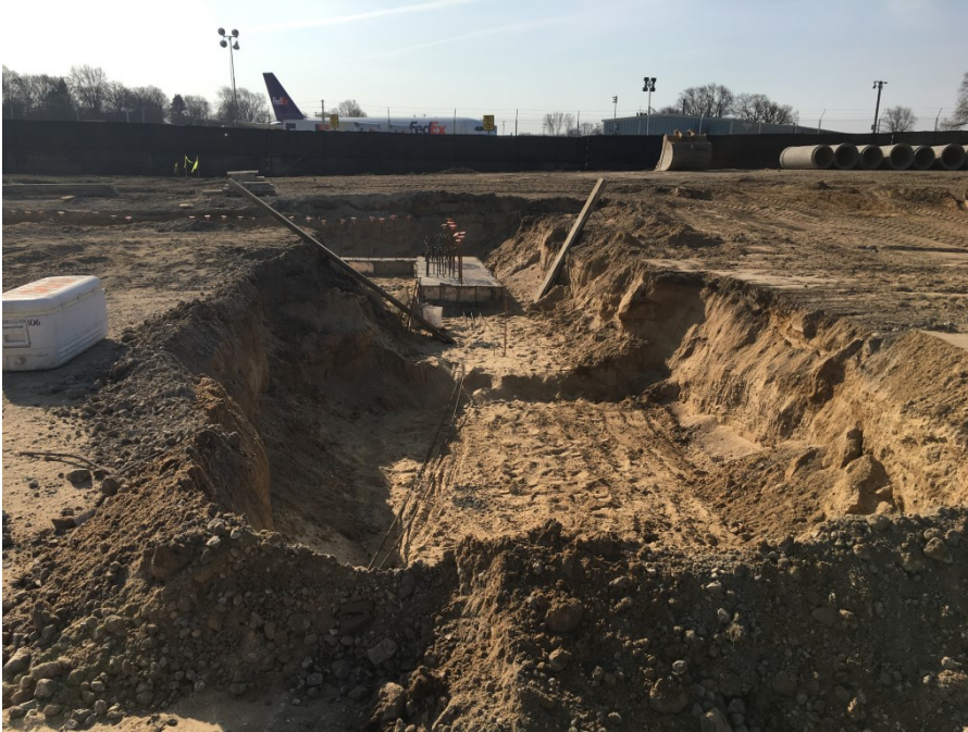
Photo 5: Footing trench looking east (4/7/21; 09:03)
