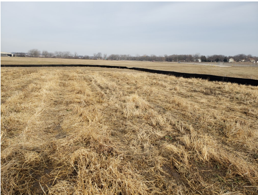
Photo 14: Soil replacement area looking north (12/15/21; 11:19)
