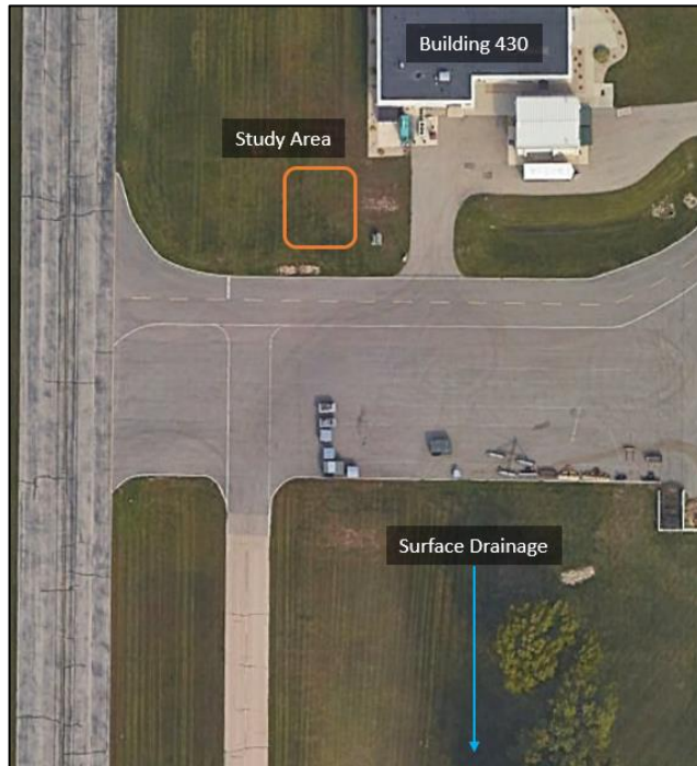
Figure 1. Aerial overview of study area.
