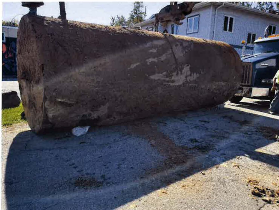
Photo of the 1 st (northern) 8,000-gallon UST following removal.
