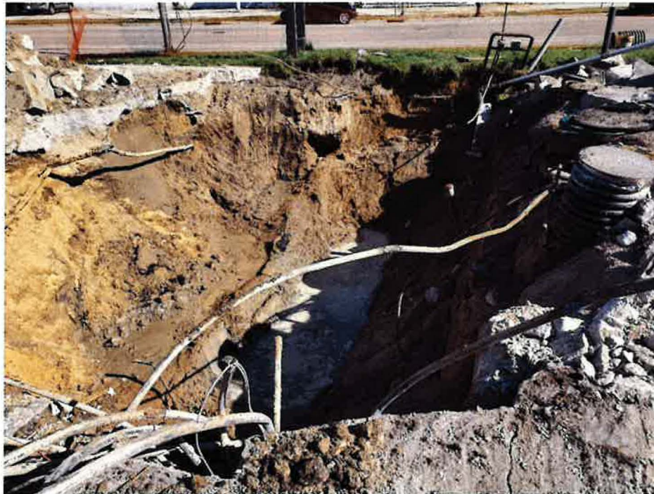
Photograph of 2 nd 8,000-gallon UL Gasoline UST following removal of the 1 st . View looking east.
