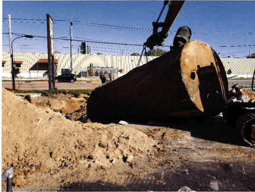
Photograph of the 2 nd (center) 8,000-gallon UST being removed
