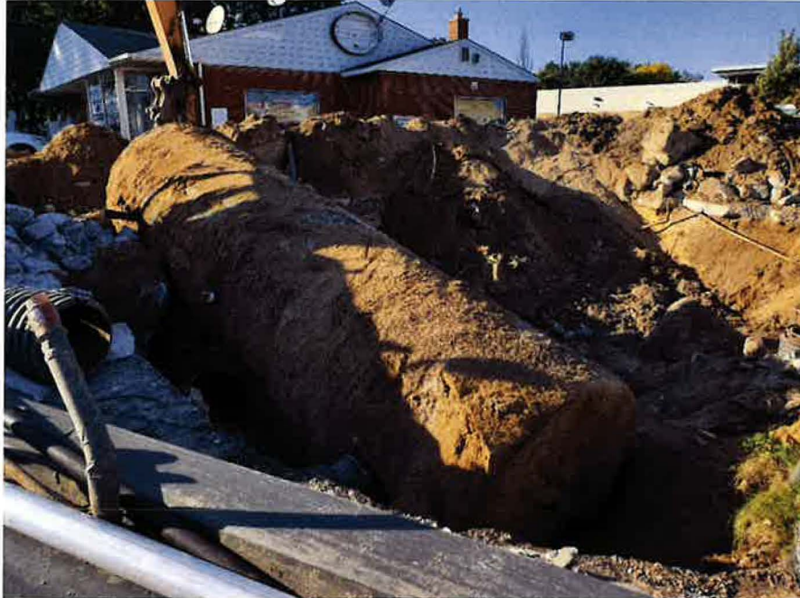
Photo of the 10,000-gallon UL Gasoline UST being removed. View looking northwest
