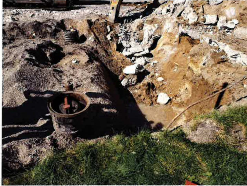
Photograph of the 1 st (northern) 8,000-gallon UL gasoline UST. Note water in the excavation.
