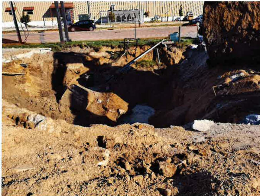
Excavation following removal of the two, 8,000-gallon ASTs.
