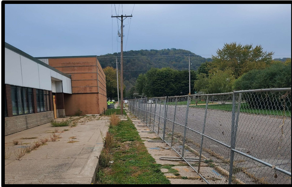
Site is Fenced and Razing Begins
