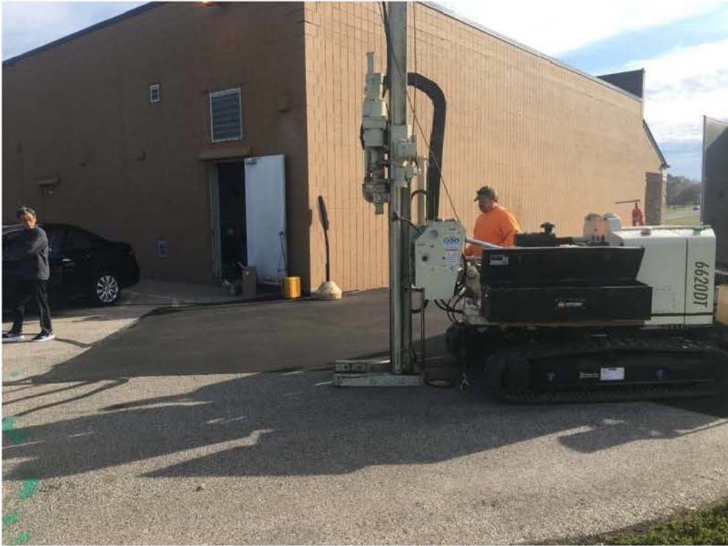
1) Photograph facing northeast of the location of soil boring P-1.
