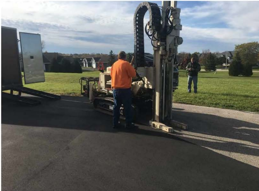
2) Photograph facing southwest of soil boring P-1.
