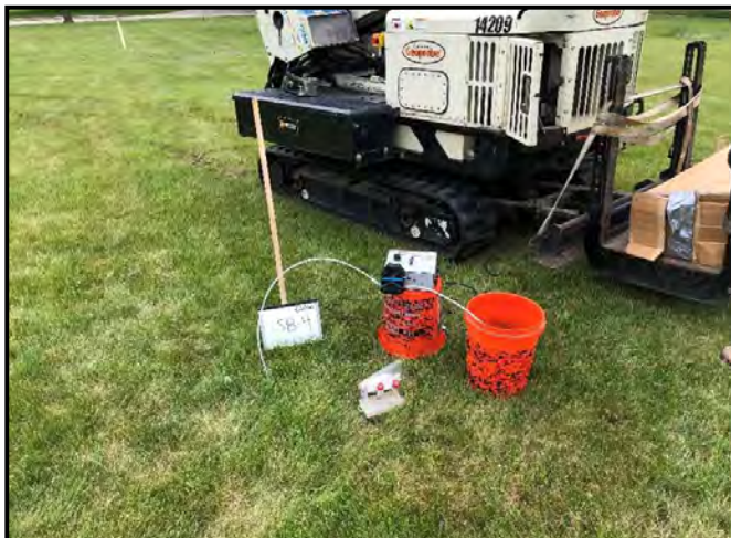
Groundwater sample collection SB-4.
