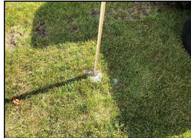
Temp well removed and soil boring SB-3 abandoned.
