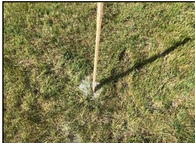
Temp well removed and soil boring SB-2 abandoned.
