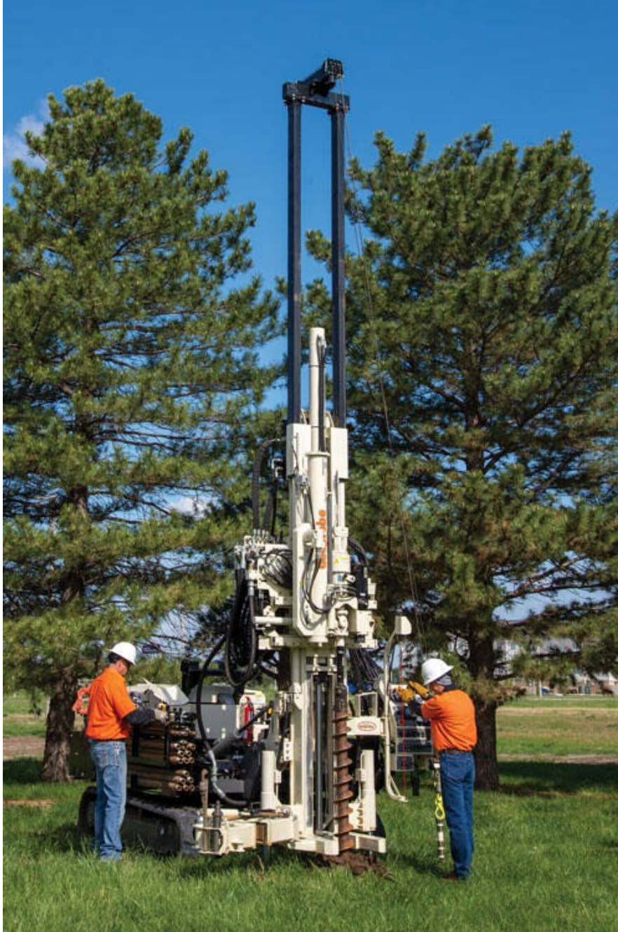
Figure 1 Monitoring well installation by hollow stem auger. Image courtesy of Geoprobe.com
