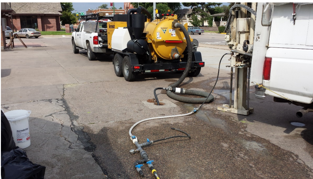
Figure 8 Vacuum extraction and in-situ injection.
