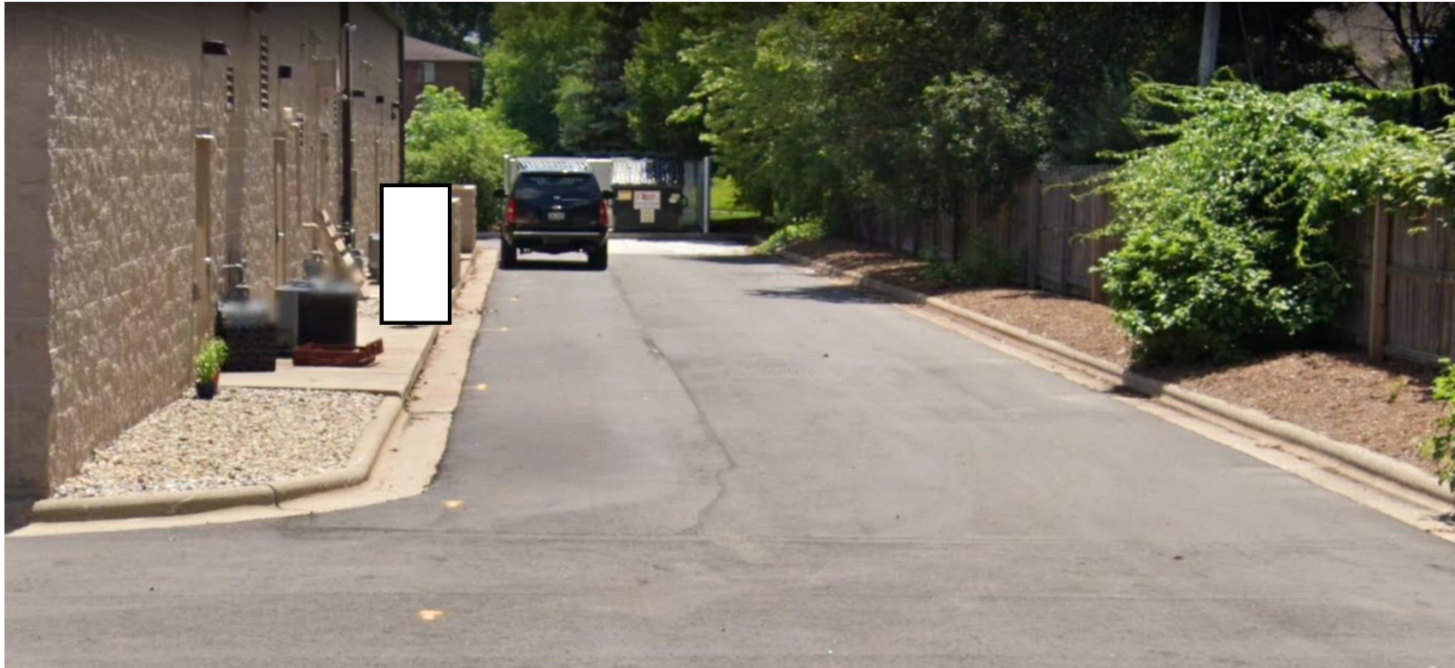
ASPHALTIC CONCRETE AND DRIVE AREA AND CONCRETE SIDEWALK PORTION OF THE IMPERMEABLE BARRIER LOOKING SOUTH FROM THE CALUMET AVENUE RIGHT-OF-WAY
