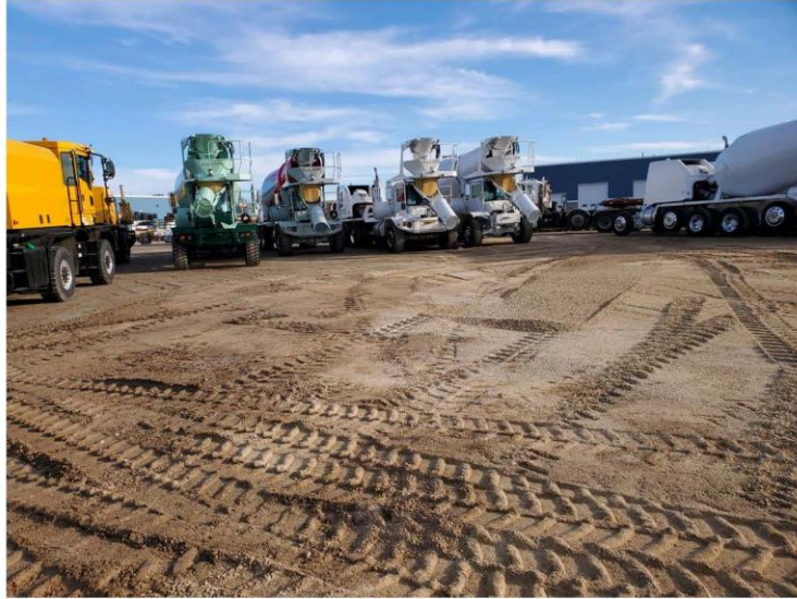
Spill area following backfill/compaction, view looking southeast
