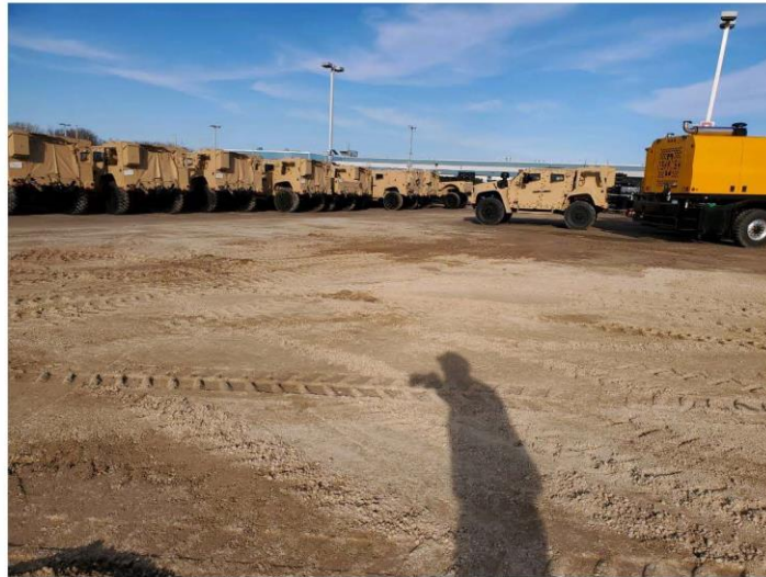
Spill area following backfill/compaction, view looking northeast
