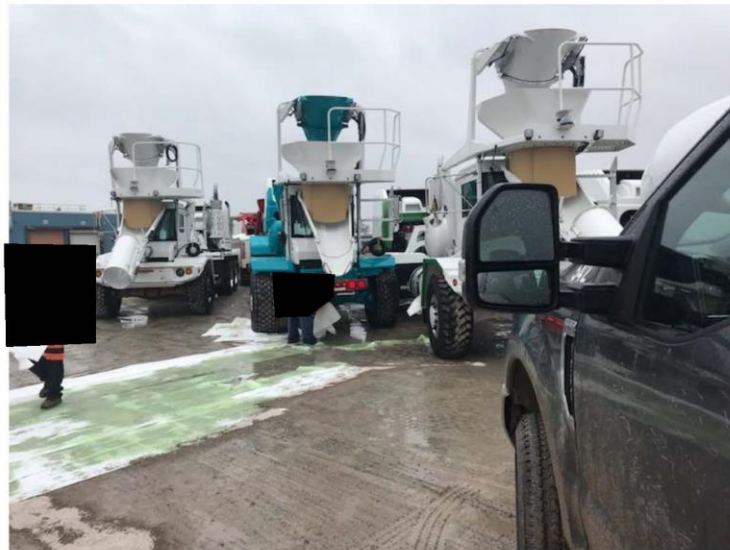
Absorbents being placed over spill.
