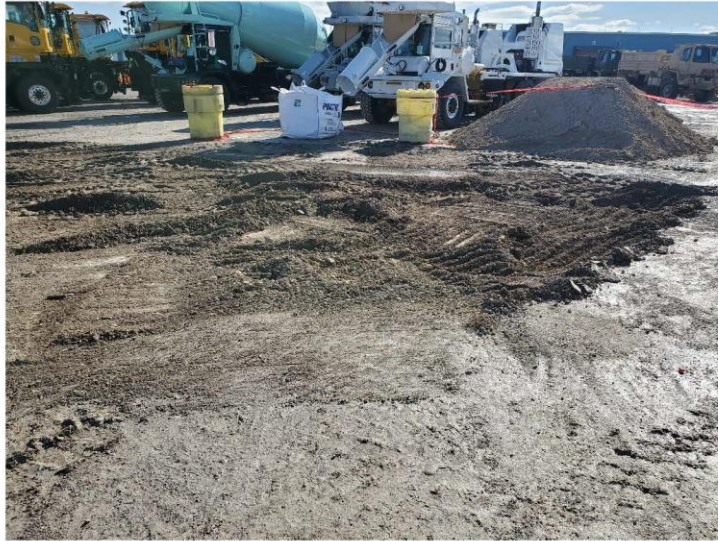
South end of scrape/excavation, view looking east
