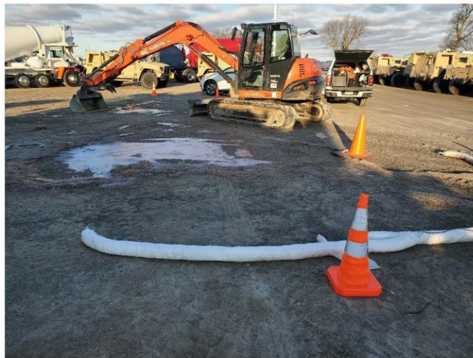
View of spill area prior to excavation, looking west
