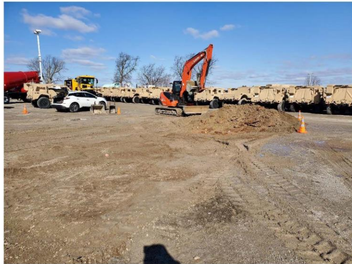
Scrape/excavation, view looking northwest
