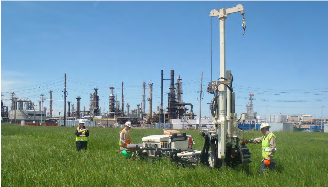
Photo 1: Setting up at SB-1.
