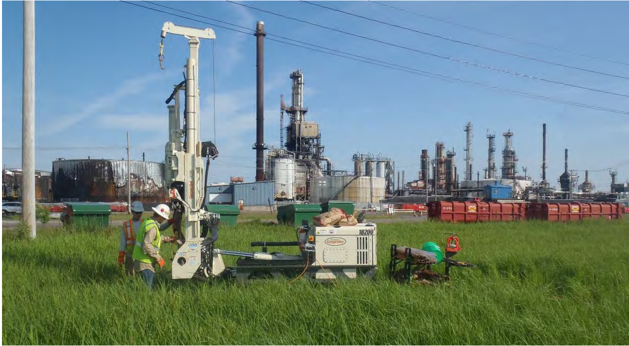
Photo 3: Advancing sampler at SB-4.
