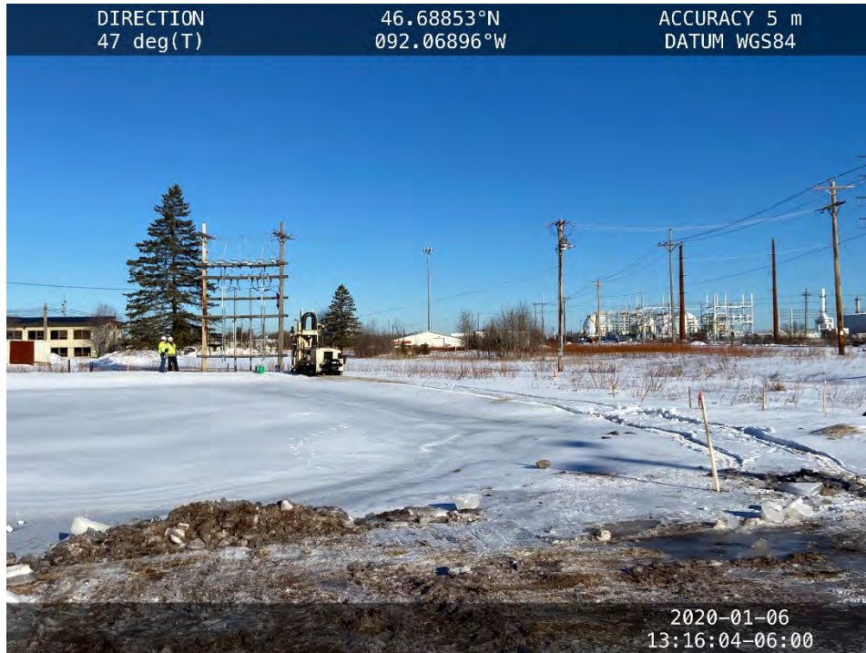
Photo 1: Preparing to drill at SB-10 on the edge of the pond.
