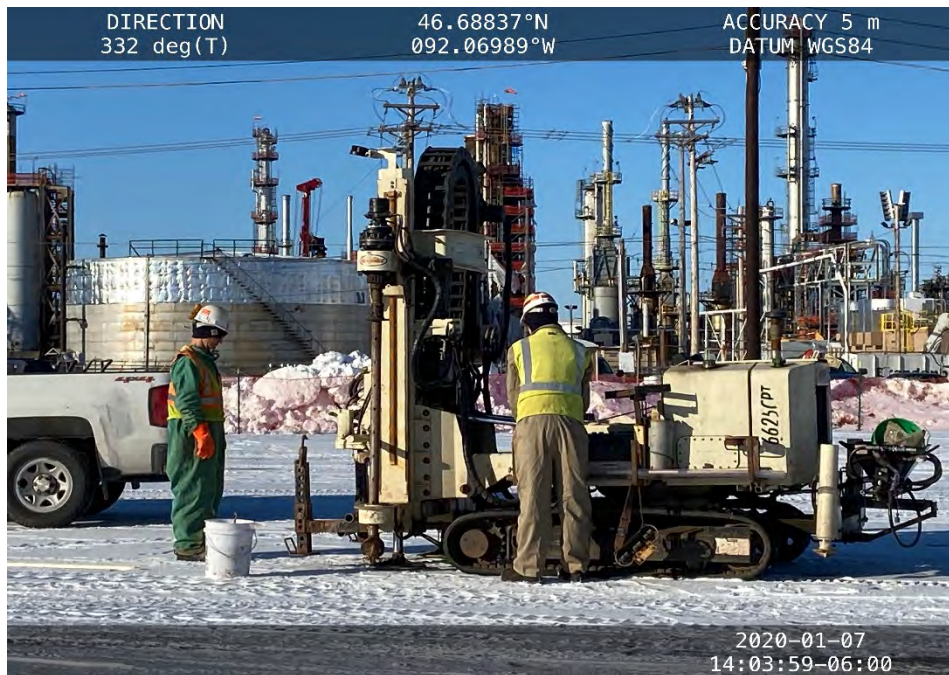
Photo 2: Drilling at SB-20.
