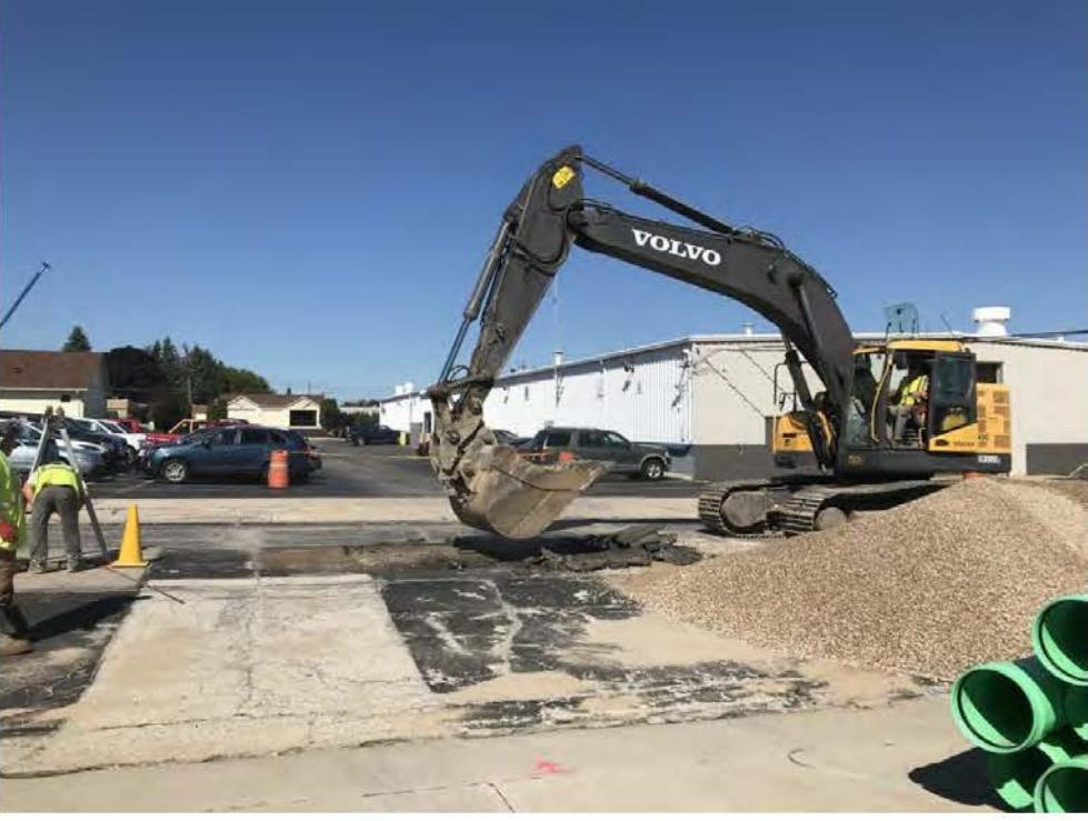
A black Volvo excavator is operating on a paved surface, removing asphalt. A worker in a yellow vest stands nearby, supervising the work. A large pile of aggregate or gravel is visible on the right side of the frame. The background shows a parking lot with several cars and a white building.                                                                                              |
