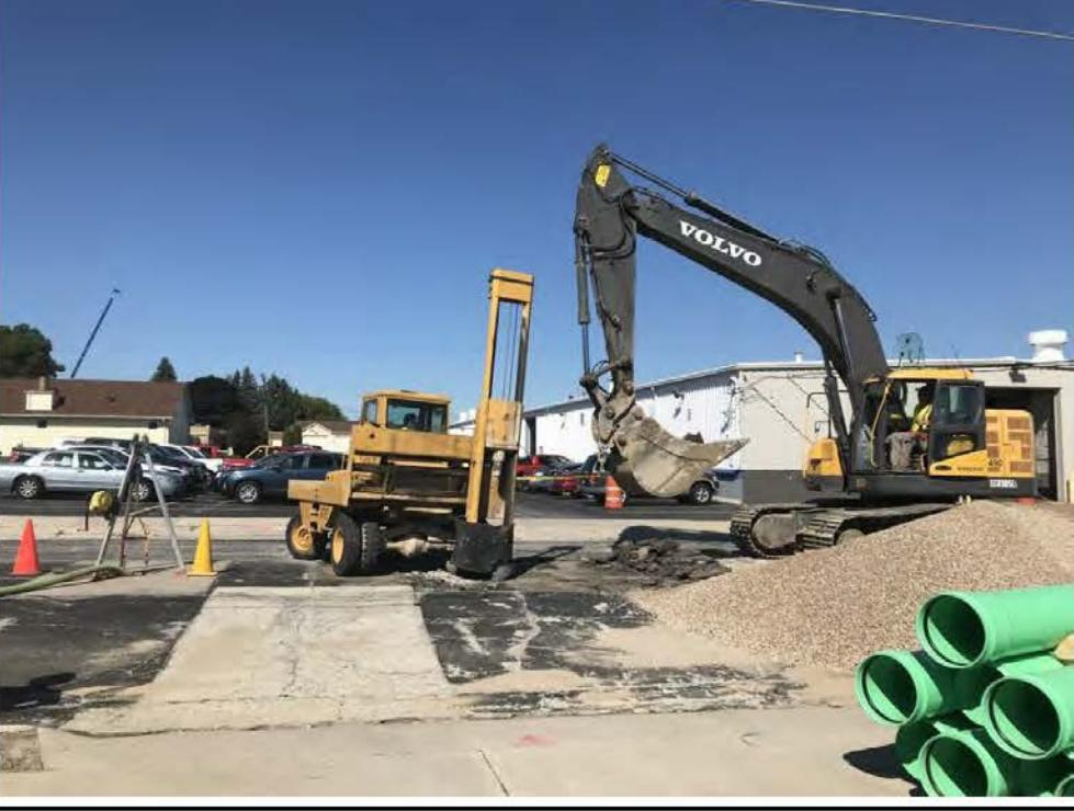
A black Volvo excavator is operating on a paved surface, breaking up concrete underlayment. A yellow utility vehicle is positioned nearby, likely to remove the broken material. A worker in a yellow vest stands near the work area. A large pile of aggregate or gravel is visible on the right side of the frame. The background shows a parking lot with several cars and a white building. |
