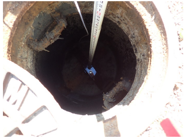
Figure 11 Survey rod and tubing set in structure to collect sample
