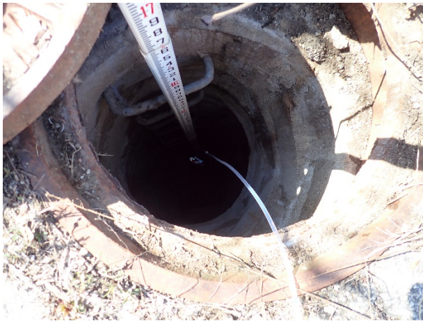
Figure 2 Survey rod and tubing set in structure to collect sample.
