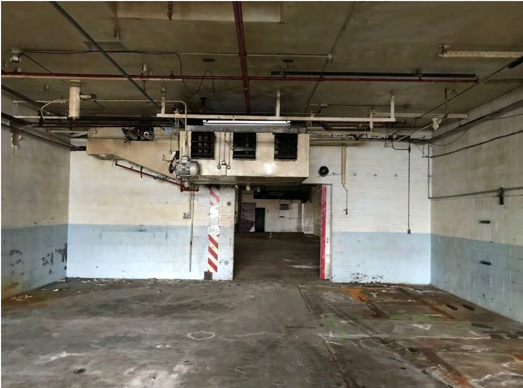
Photo 3: Solvent cleaning room looking south
