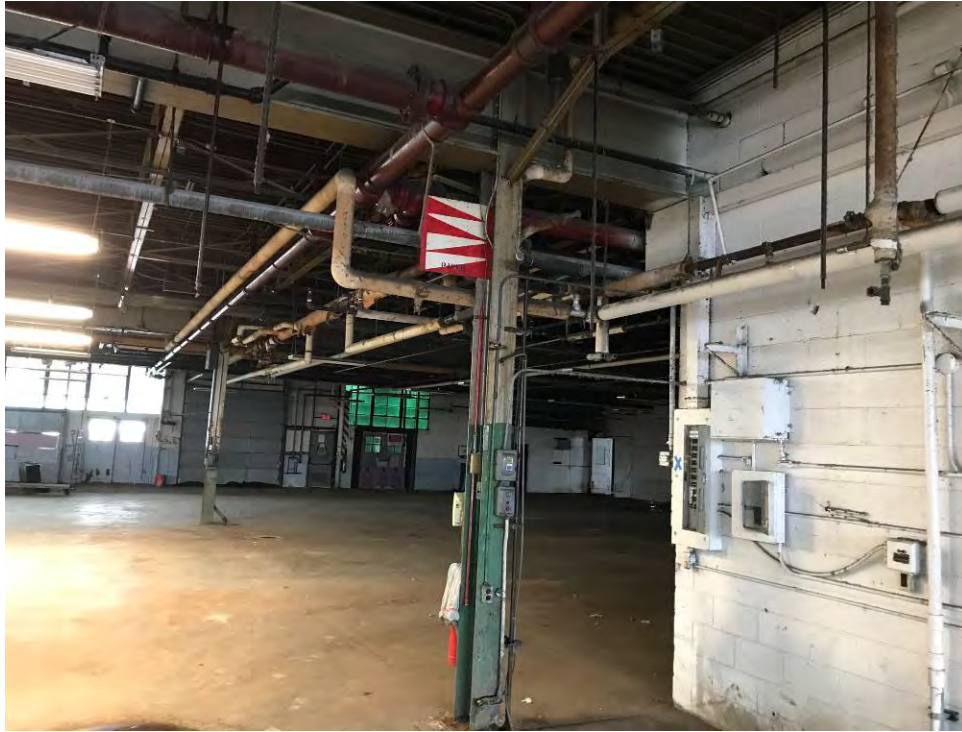
Photo 5: Looking south from southeast corner of dry-cleaning room
