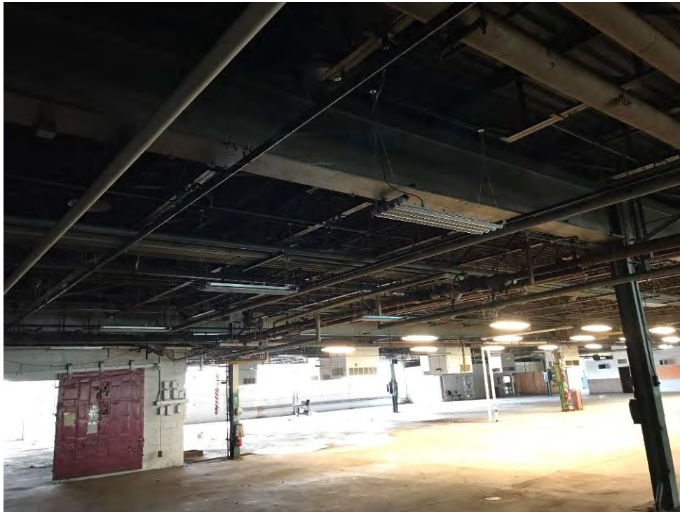
Photo 6: Looking northeast from Area of SB #7
