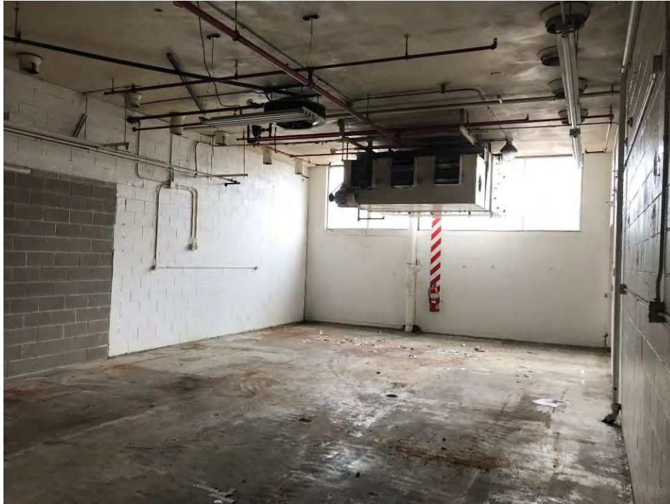
Photo 1: Dry-cleaning room looking north
