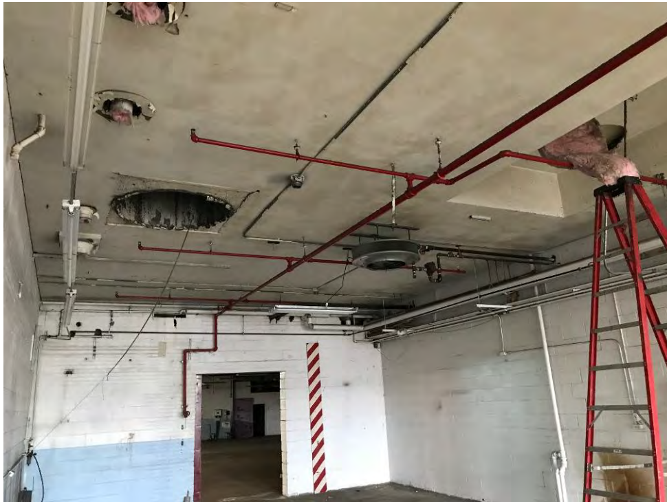
Photo 2: Dry-cleaning room looking south
