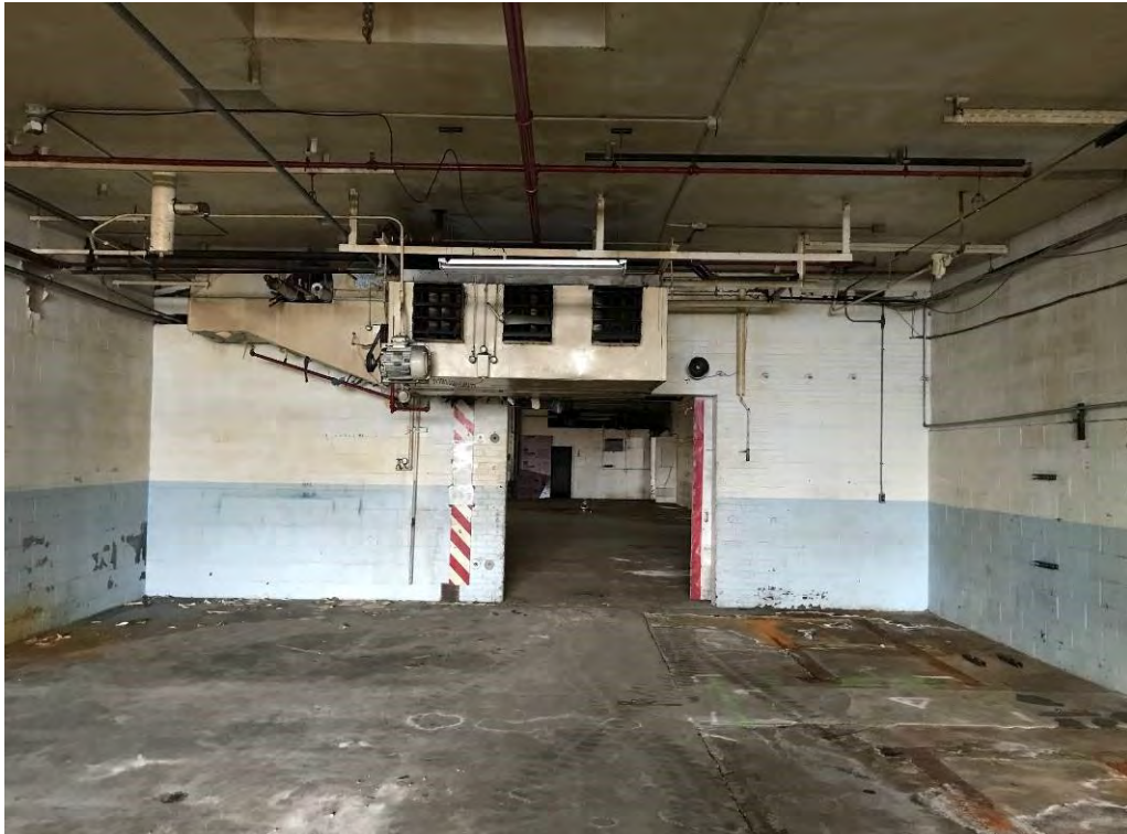
Photo 3: Solvent cleaning room looking south
