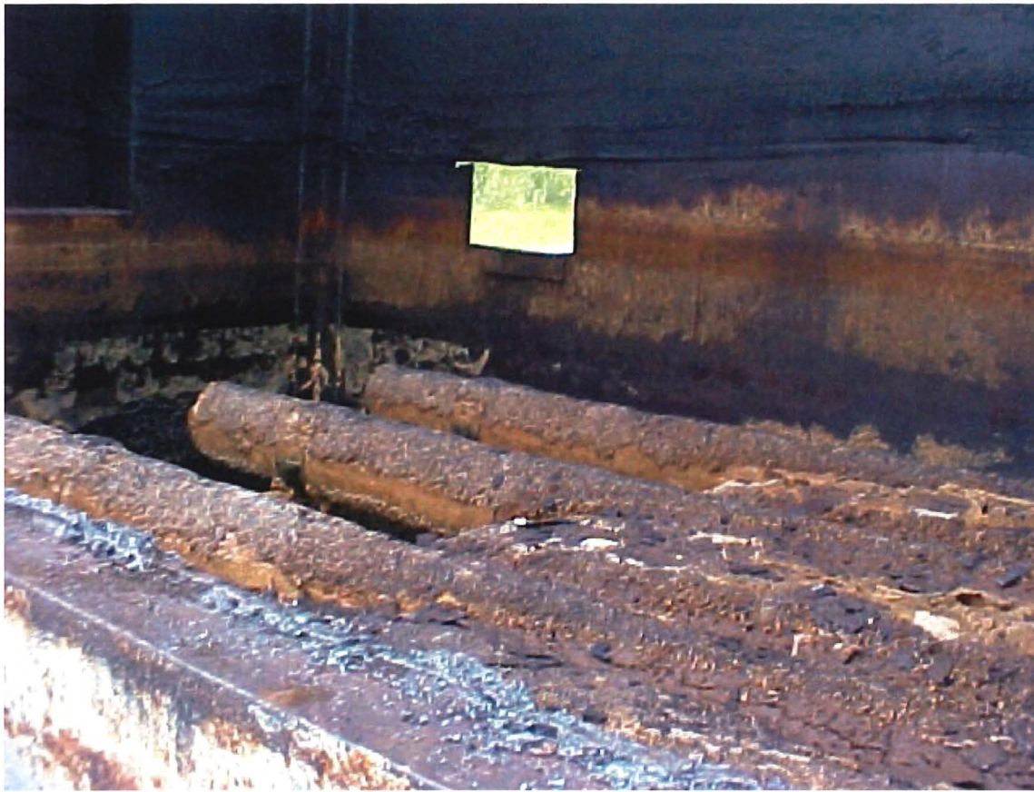
Inside of small evaporator prior to cleaning.
