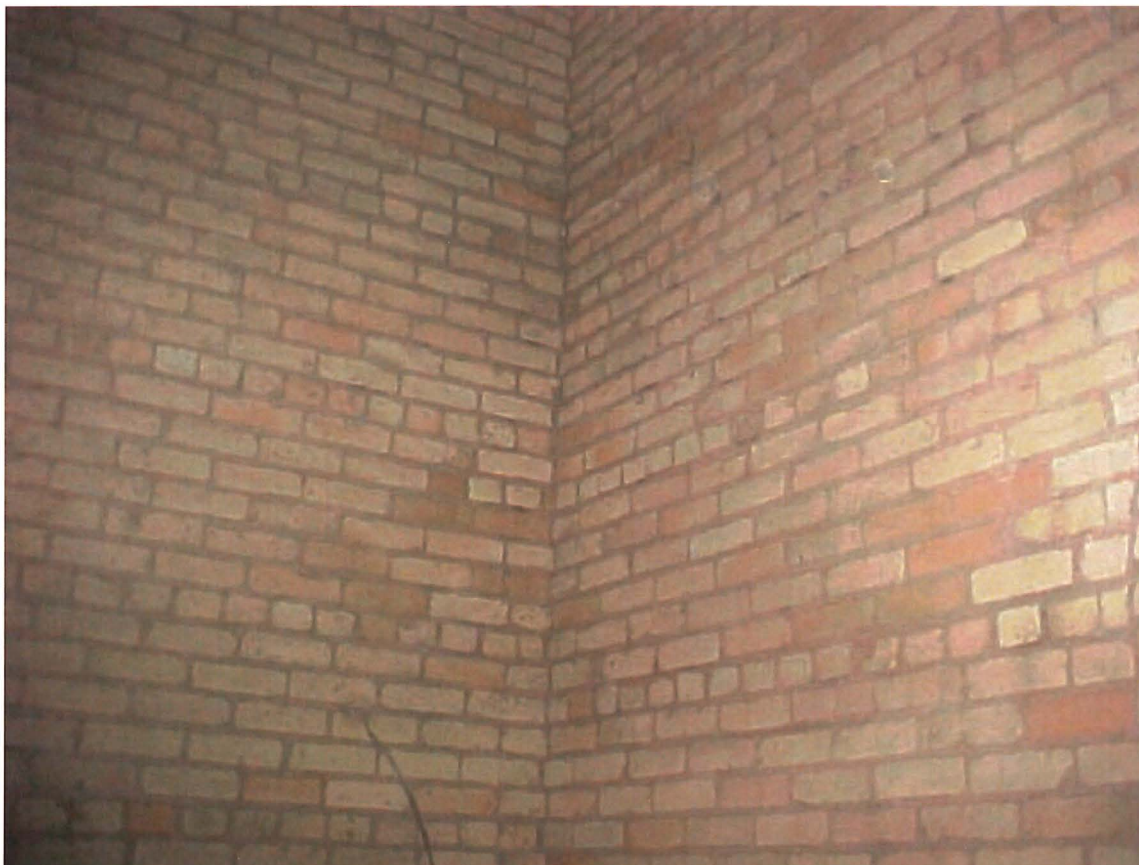
Southwest corner of treating building after sandblasting
