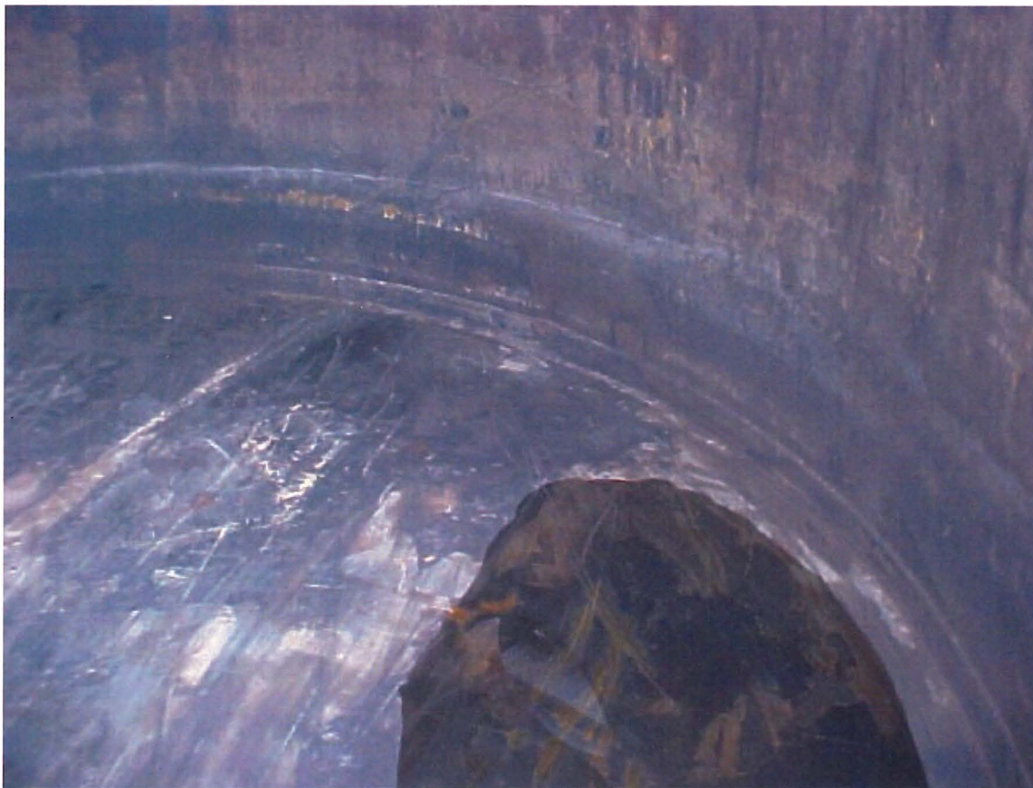
Inside of F tank after pressure washing.
