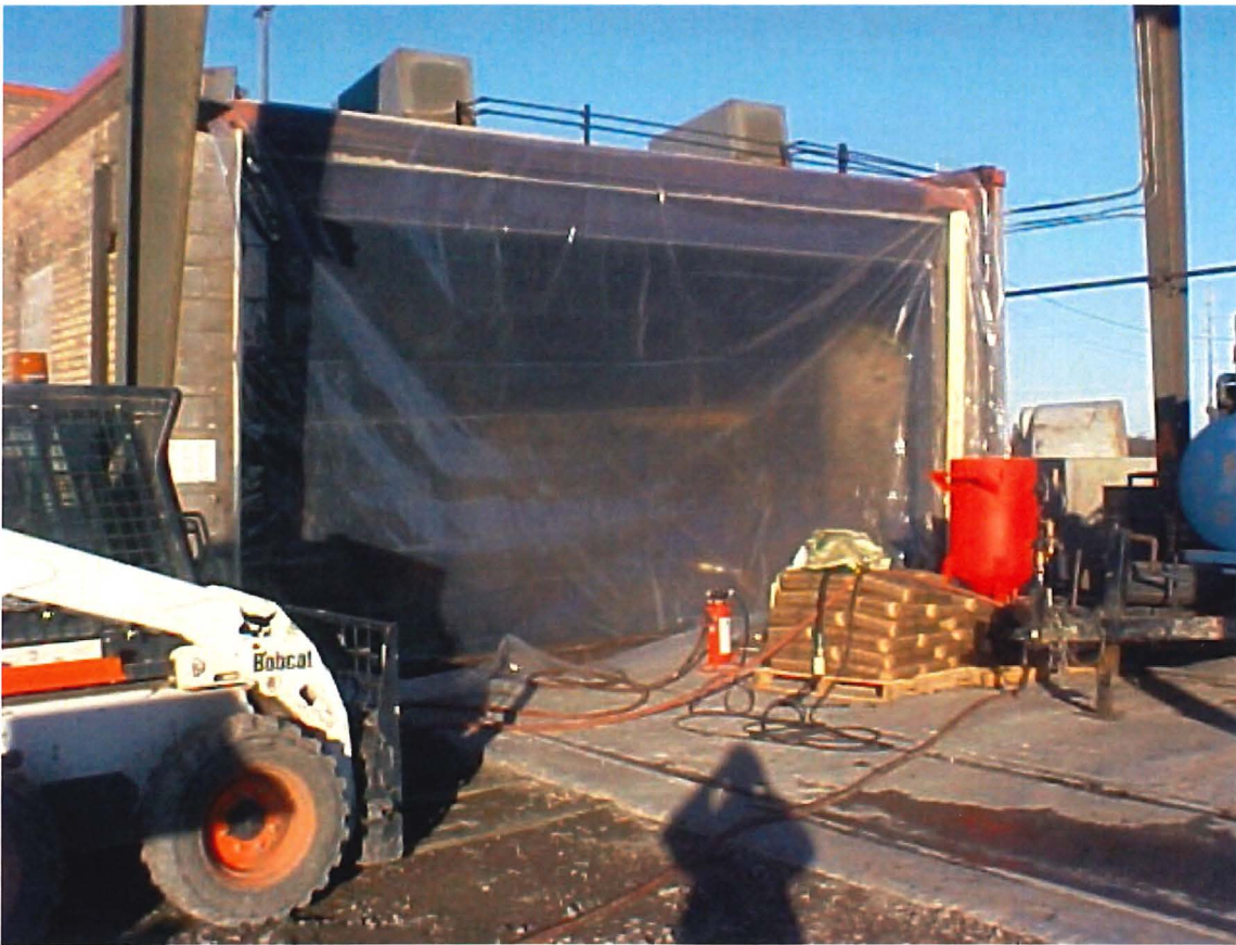
Example of cylinder door area isolated off prior to sandblasting.
