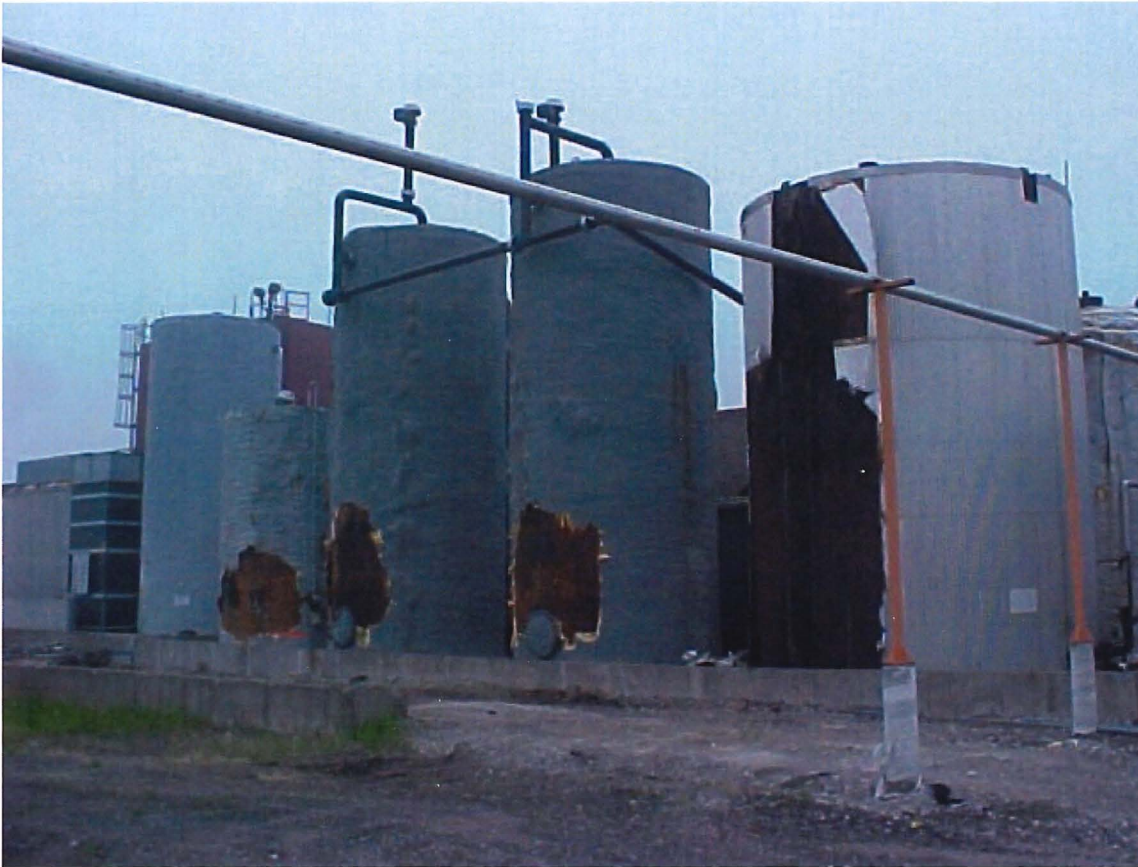
Tank farm after first week of work.
