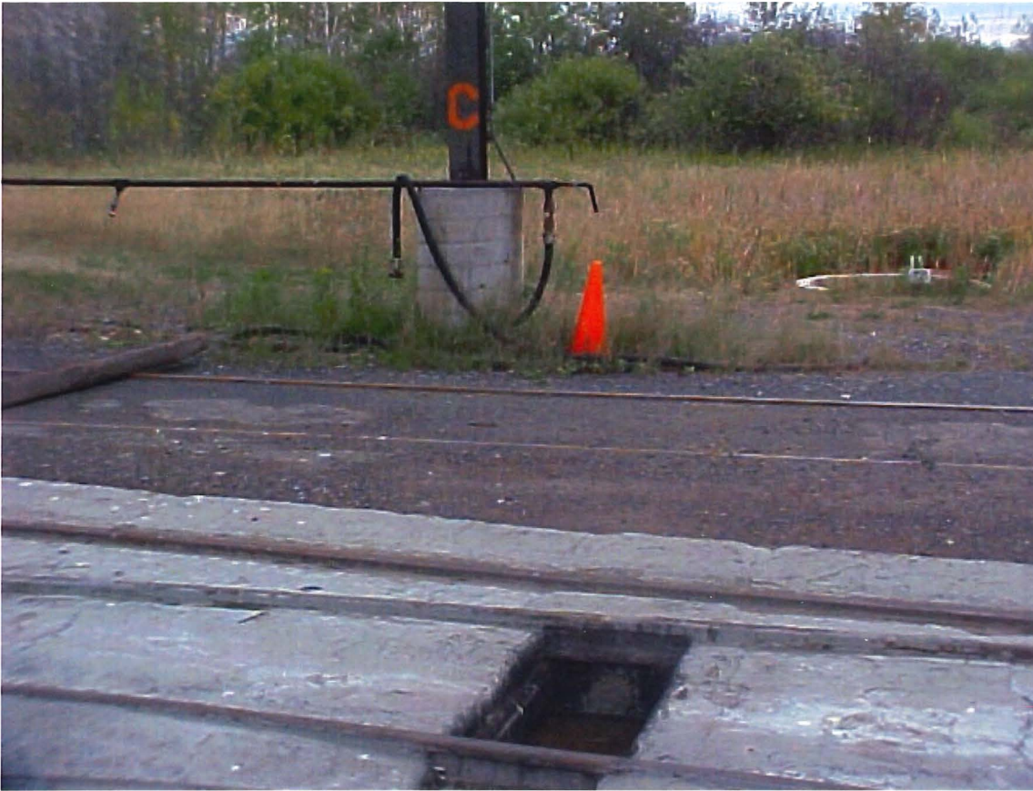
Example of drain line closed off in basin after pressure washing drain line.
