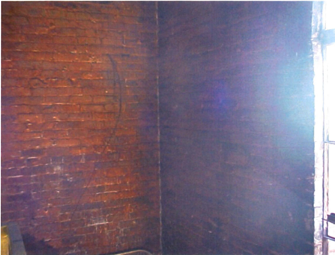
Southwest corner of treating building prior to sandblasting
