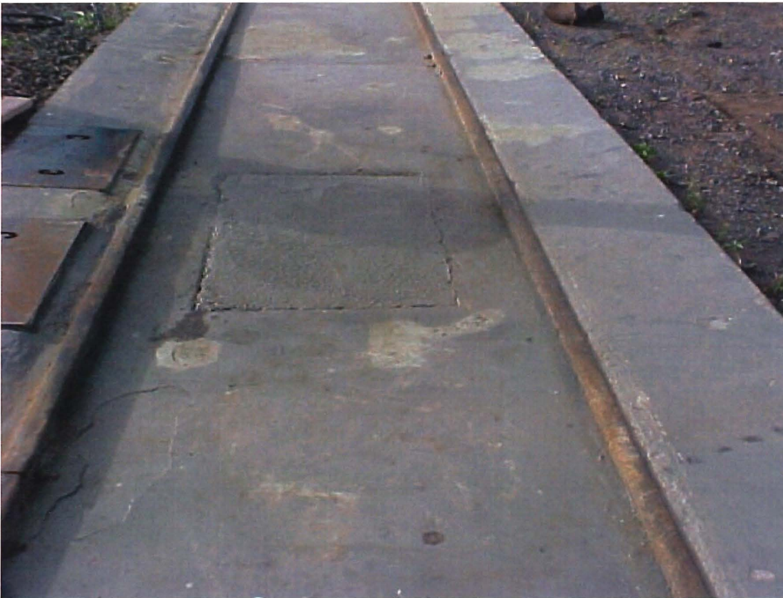
Catch basins filled with concrete to same level as drip pad.
