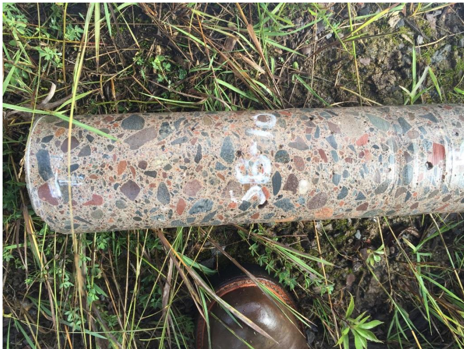
SB-10 Concrete Core
