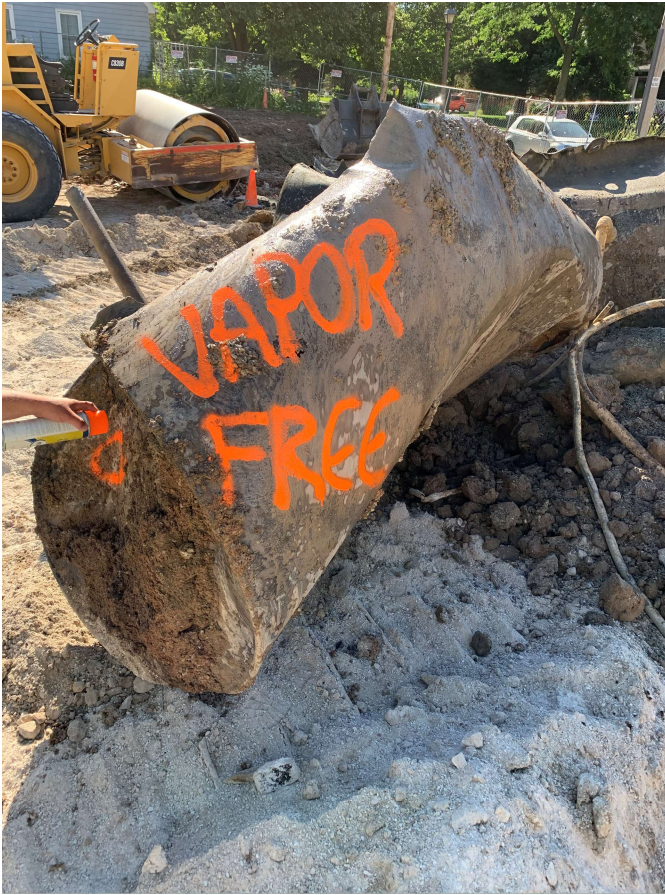
South Tank Removed with North Tank in Background
