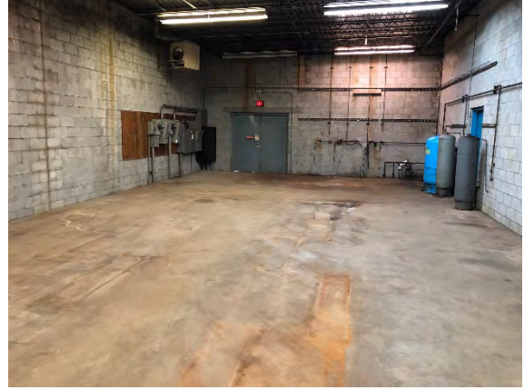
Photo 4 – View of the garage storage area on the subject property.
