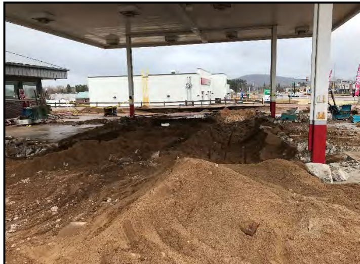
Gasoline canopy - islands and piping removed
