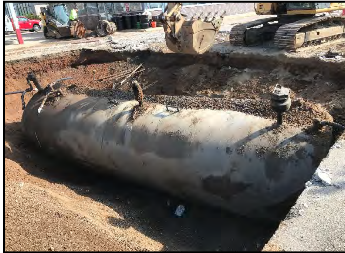
Pulling 10,000 gallon unleaded UST
