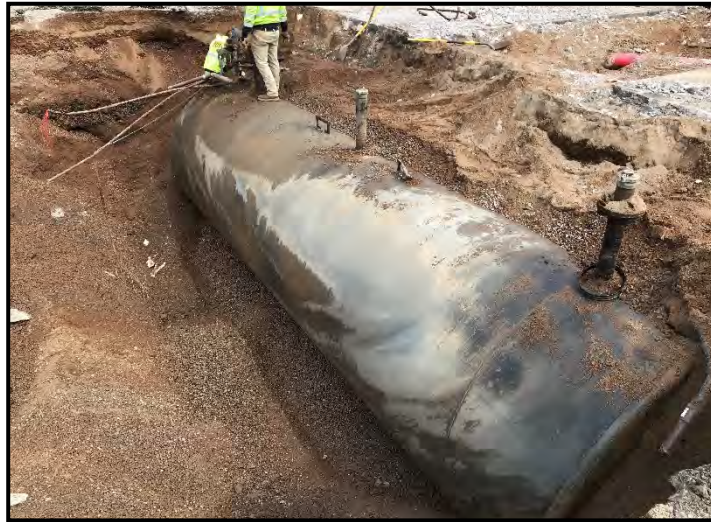
Pulling diesel UST
