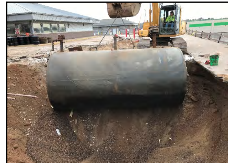
Pulling 6,000 gallon unleaded UST
