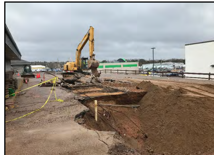
Removing diesel piping and islands
