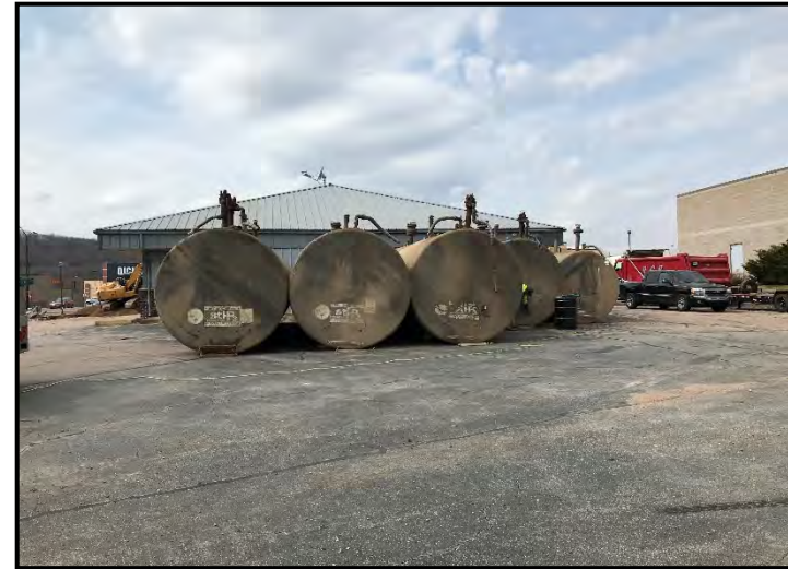
All USTs removed
