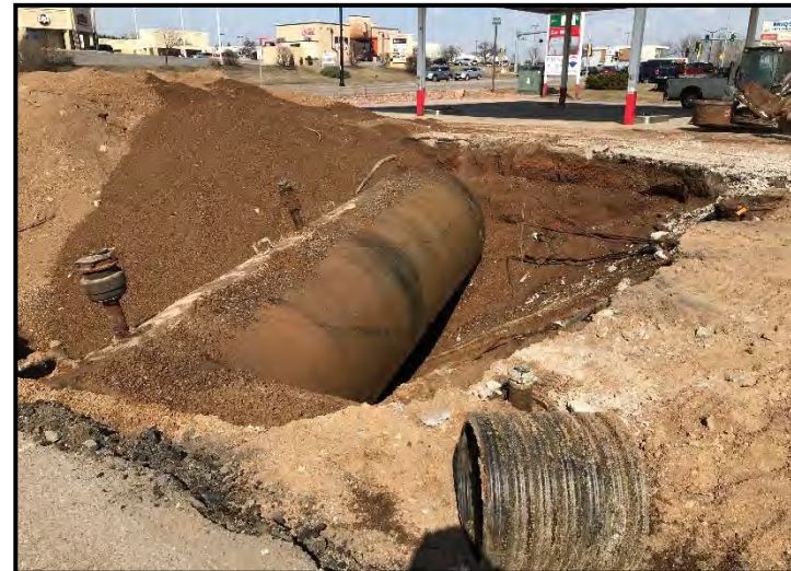
Pulling 10, 000 gallon unleaded UST
