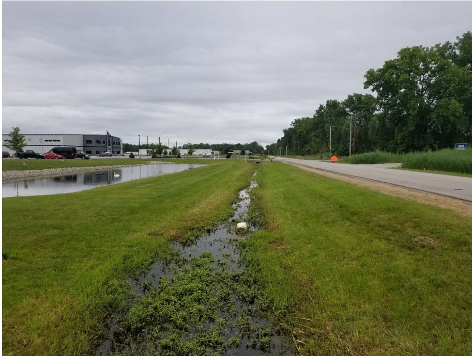
PHOTOGRAPH OF DITCH LINE EXTENDING SOUTH FROM THE SITE AND WATER DETENTION POND ON THE SOUTHERN ADJOINING PROPERTY
