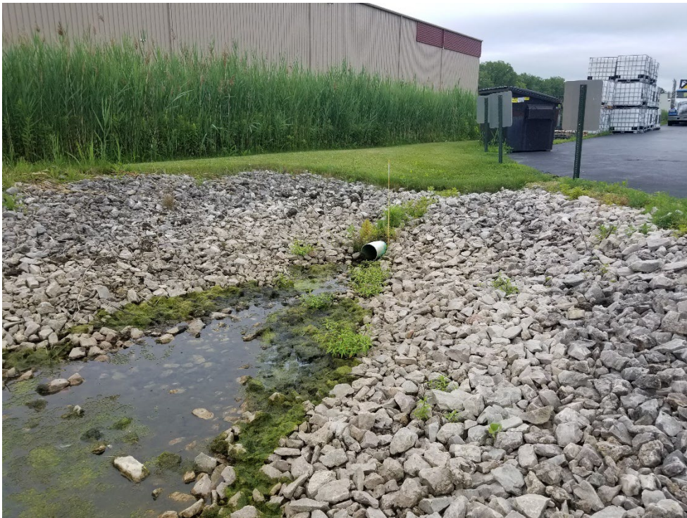
PHOTOGRAPH OF HIGHWATER POND OUTFALL AND DRAINAGE SWALE WITH OVERGROWN VEGETATION ALONG SOUTHERN BOUNDARY OF THE SITE
