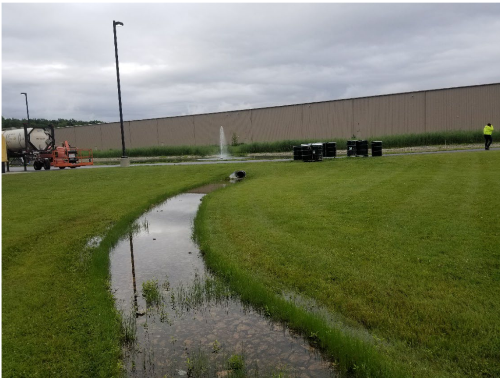
PHOTOGRAPH OF DRAINAGE SWALE EXTENDING SOUTHEAST TOWARD POND
