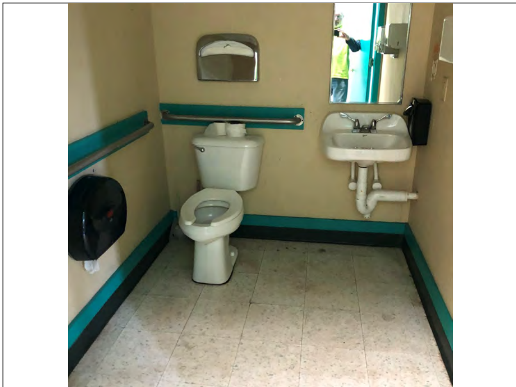
Photo 12: Restroom in the self-serve laundry mat area.
