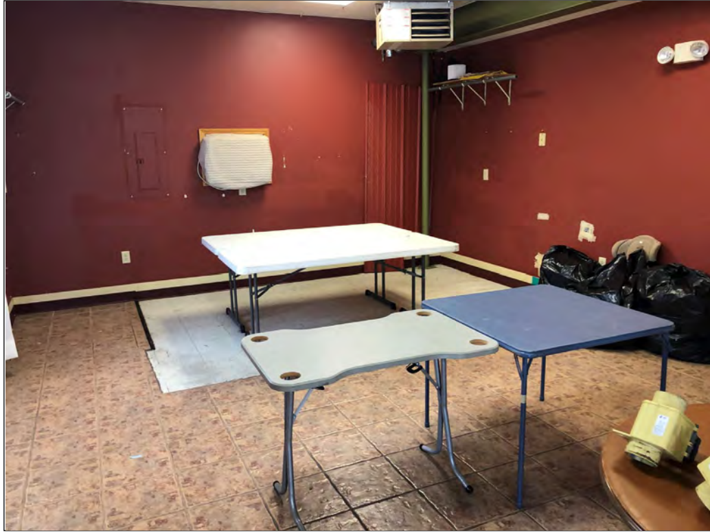
Photo 15: Office area space on the west side of the building.
