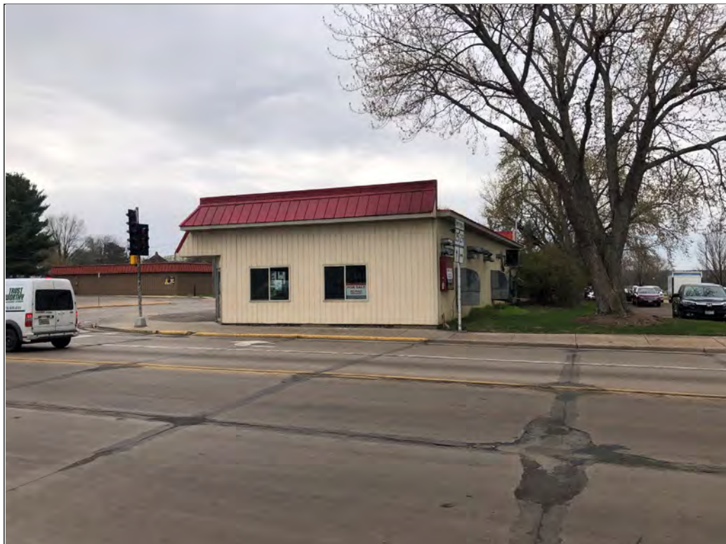
Photo 4: East side of the building adjacent to South Broadway Street.
